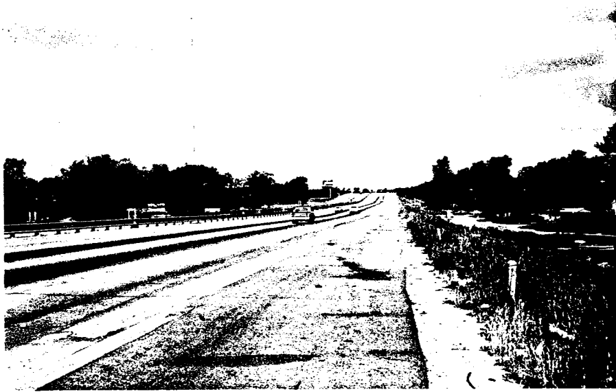
View Downstream From Station 1
