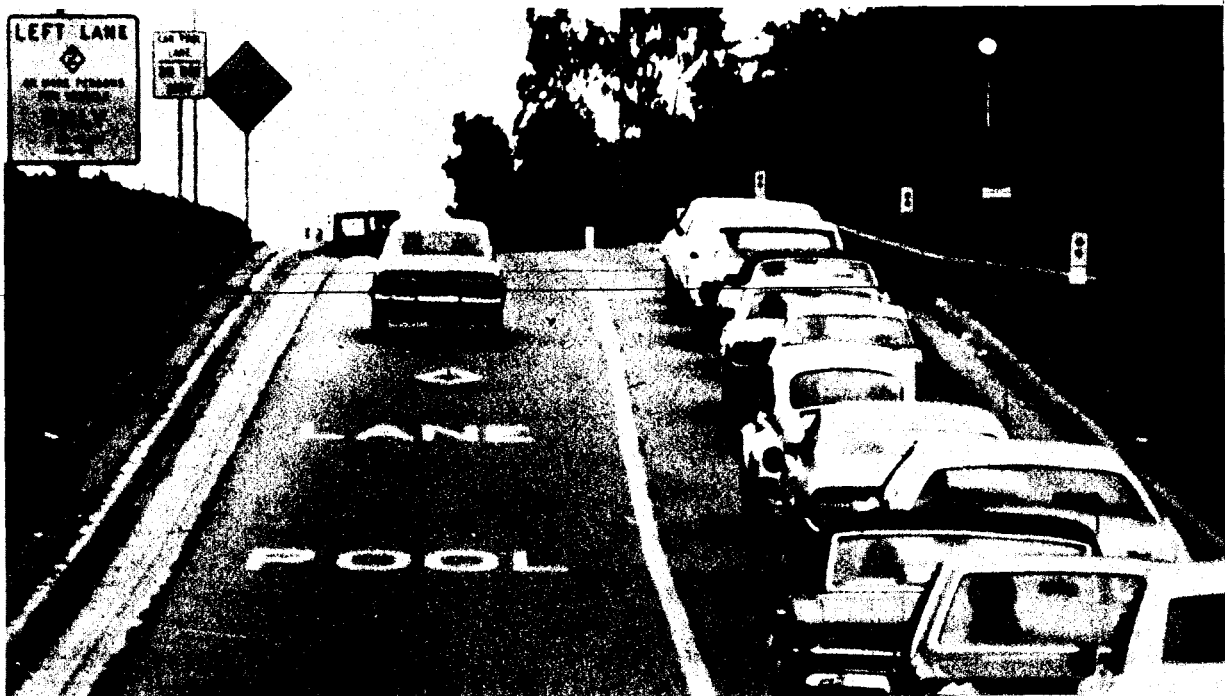
Priority entry provides a special lane for buses and/or carpools. In Minneapolis (top), buses enter the freeway ahead of vehicles queued at a ramp signal, while carpools enter the Santa Monica Freeway (bottom) in Los Angeles via a lane that bypasses cars waiting at a ramp signal.
