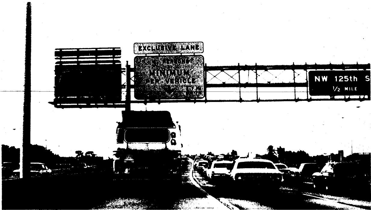
Concurrent flow reserved lanes are designated adjacent to the median using signs and markings. The Santa Monica Freeway (top) in Los Angeles utilized an existing lane while the I-95 (bottom) concurrent flow lane in Miami was added to the freeway.
