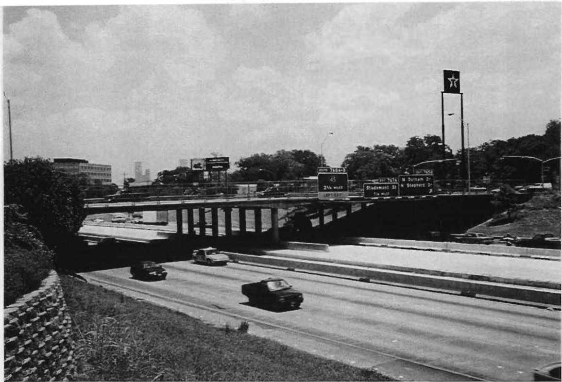
Figure 2. TC Jester Overpass (I 10W)
