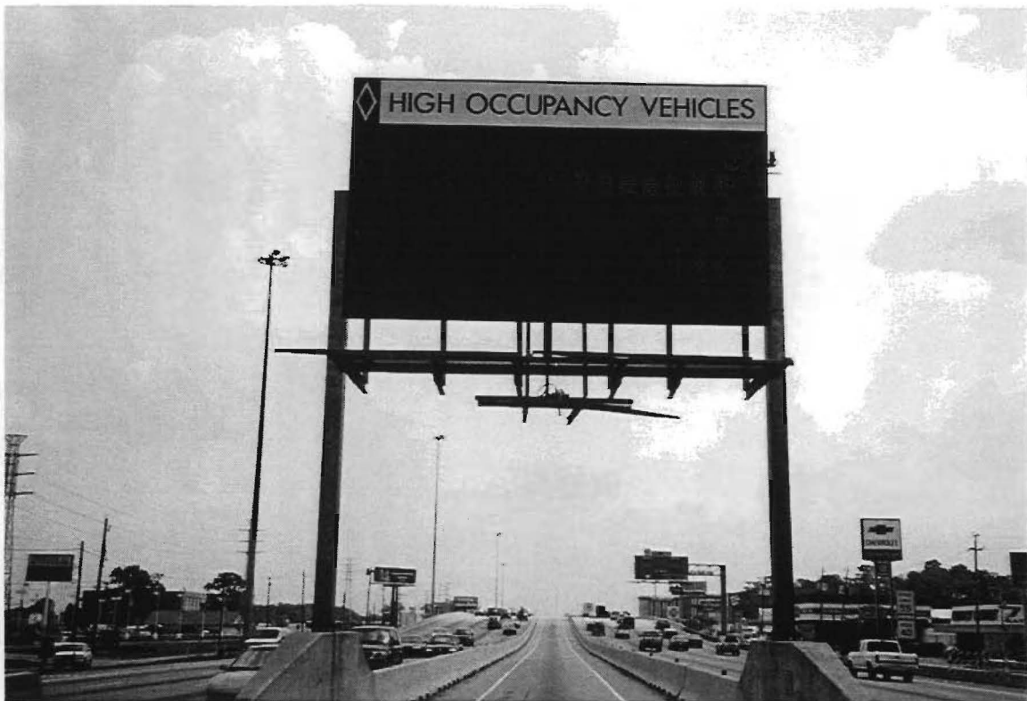
Figure 5. HOVL Overhead CMS Structure (I 10 West of I 610)
