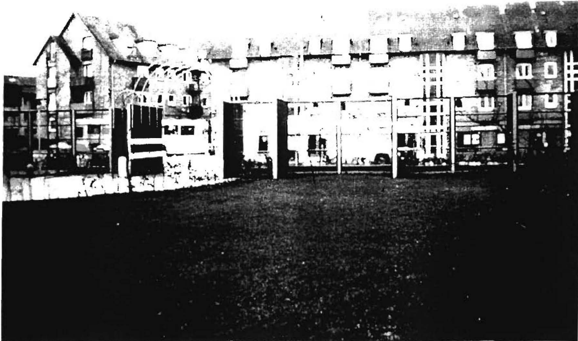
Figure 15: Transparent Noise Barrier in Soborg Hjøvedgade, Denmark, 6 m (19.68 ft.) Reinforced Glass Framed in Wood. (Copyright Hans Bendtsen. Road Directorate Denmark Ministry of Transport, Traffic Safety and Environment)
