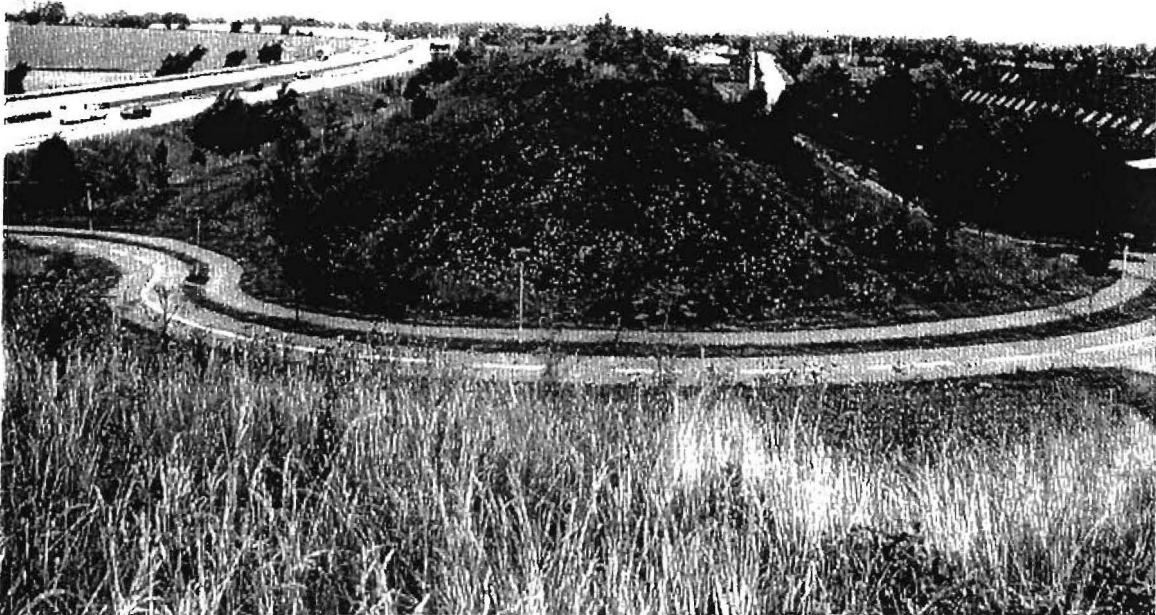
Figure 3: Earth Berm Planted with Native Grass, Shrubs, and Trees located between Highway and Adjacent Neighborhood Near Copenhagen (Copyright Hans Bensten. Road Directorate Denmark Ministry of Transport Traffic Safety and Environment)
