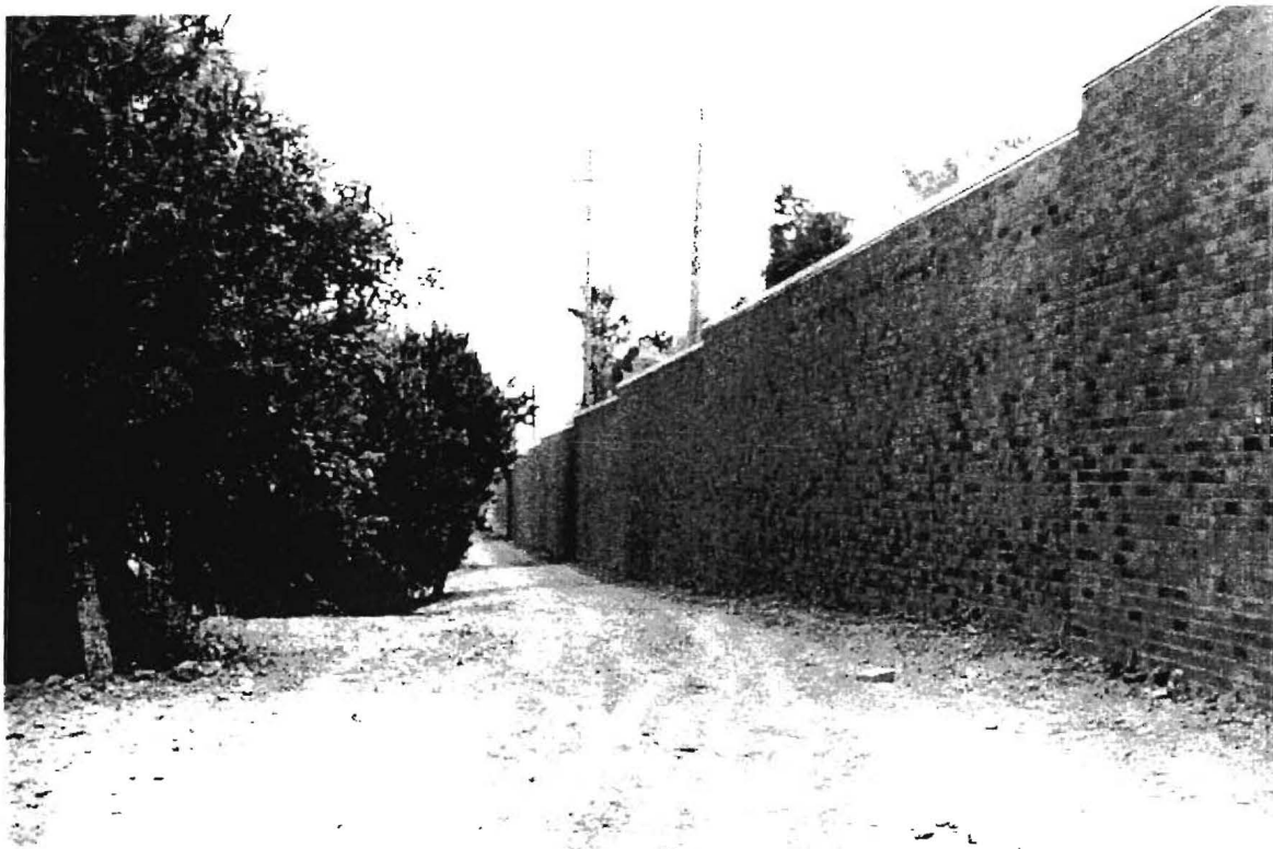
Figure 12. Reinforced Concrete Block, 4" Half-high Units with Founders Finish and Limestone Cap (Michigan DOT)
