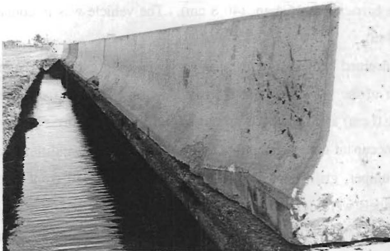
Figure 13. Limited-slip concrete barrier connection test 1959A-1 installation.
