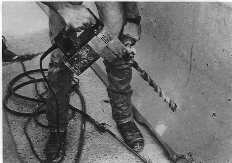
Figure 4. Drilling of pavement.
