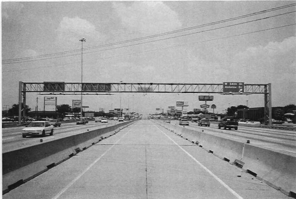
Figure 3. Overhead Sign Structure East of W. 34th Street (US 290)
