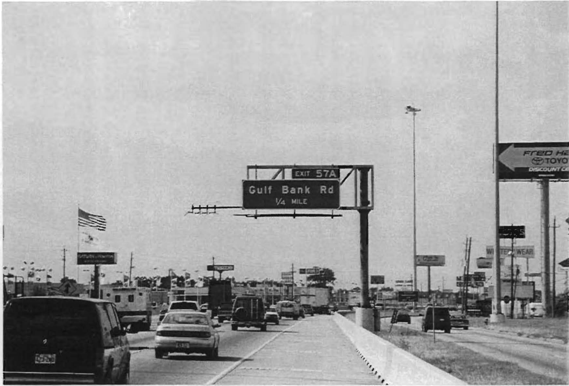
Figure 6. Side-Mount Sign Structure at N. Shepherd (I-45 NB–Gulfbank Exit)
