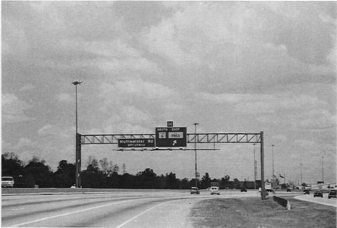
Figure 4. Overhead Sign Structure East of FM 1960 (US 290 WB Mainlanes)
