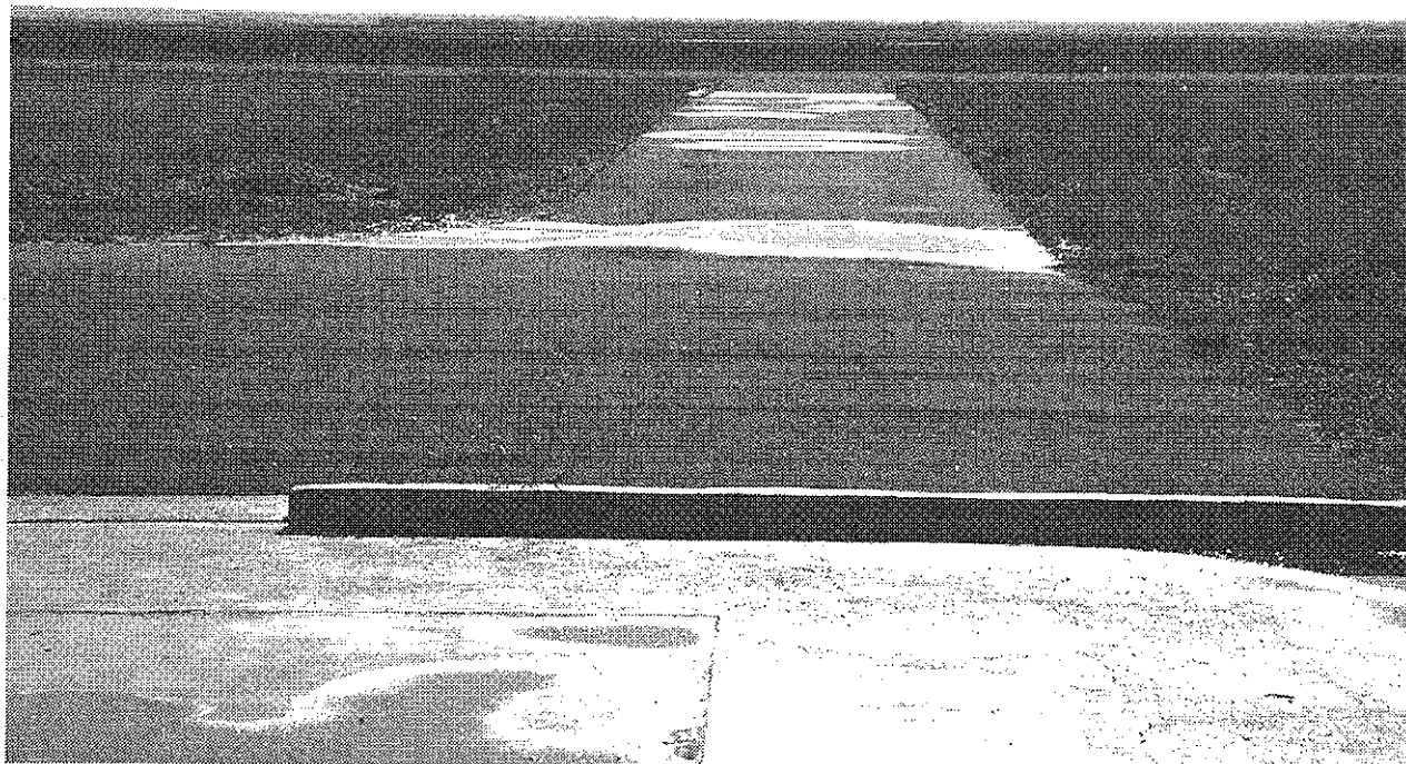
FIGURE 13. Example of a Stub Taxiway
