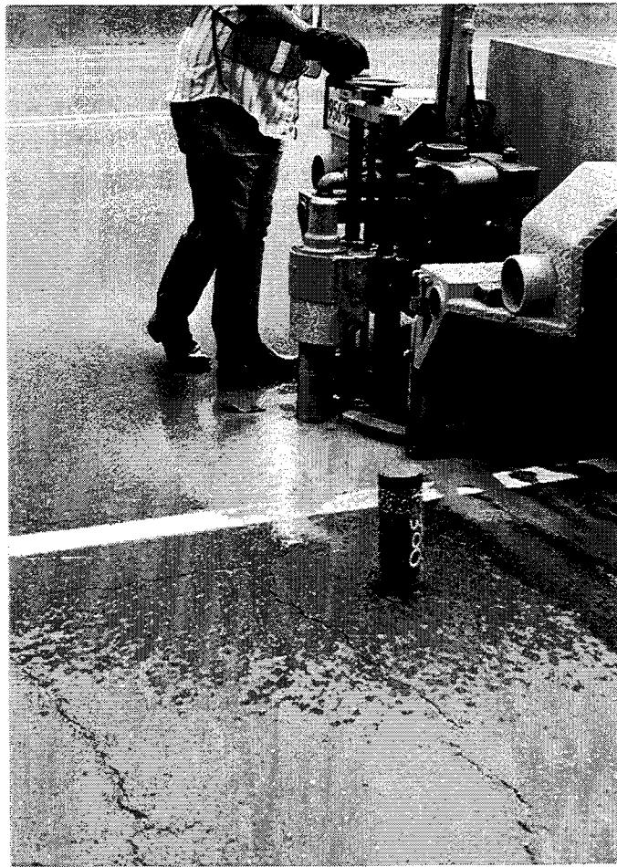
Figure 4. Ground Truth Testing on US 190 showing two asphalt layers and stabilized base.
