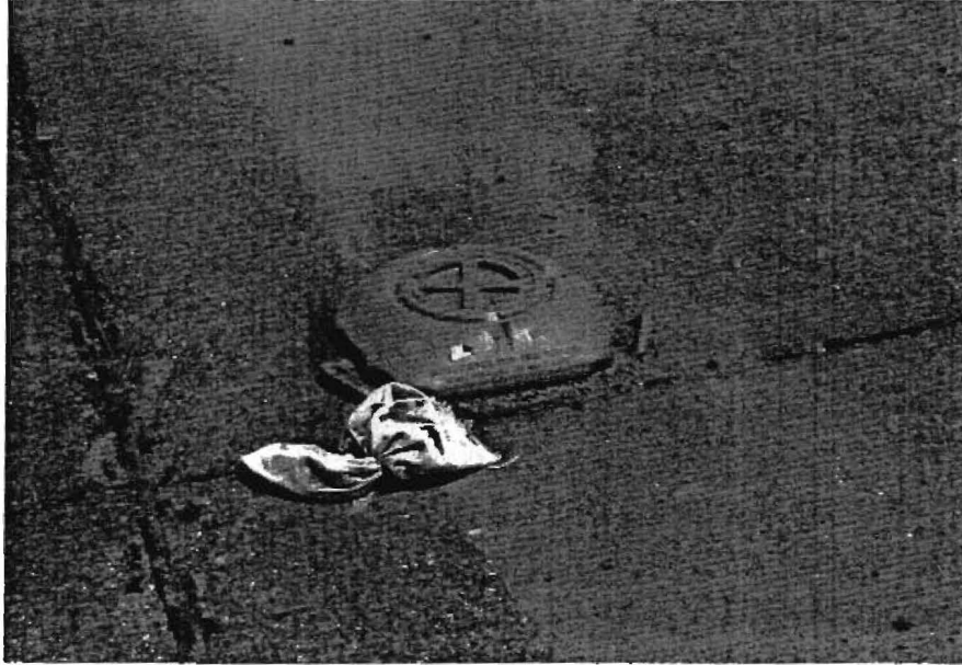
Base moved 2 in down
