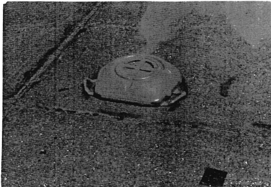
Base moved 4 in down
