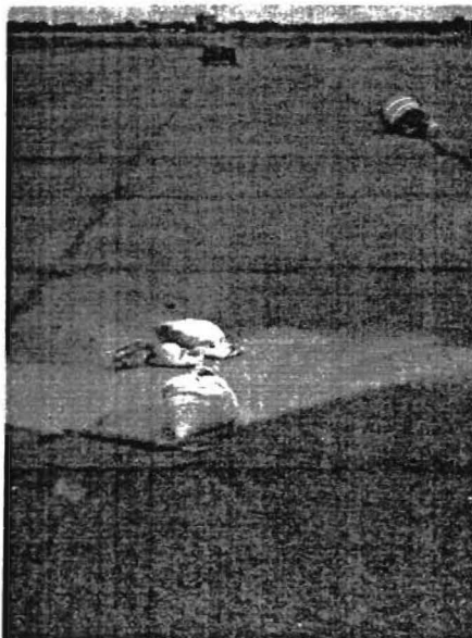
Figure 41. Test site before and after test 1817-12
