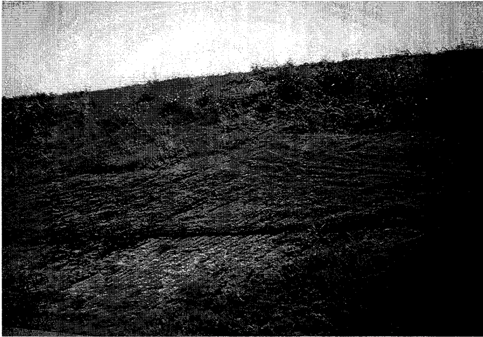
Figure 43. Slope with No Initial Erosion Control Protection
