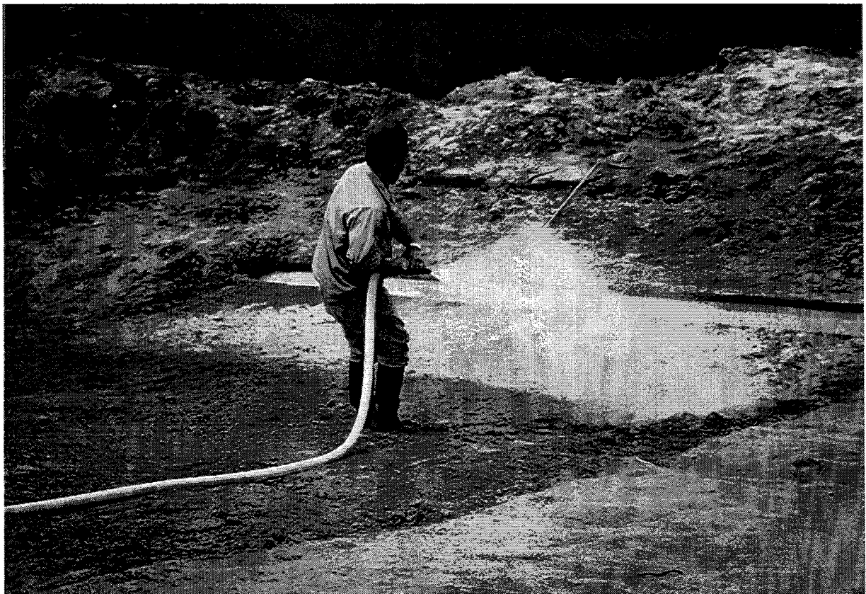
Figure 10. Installation of AIRTROL® Plaster on 2:1 and 3:1 Sand and Clay Slopes
