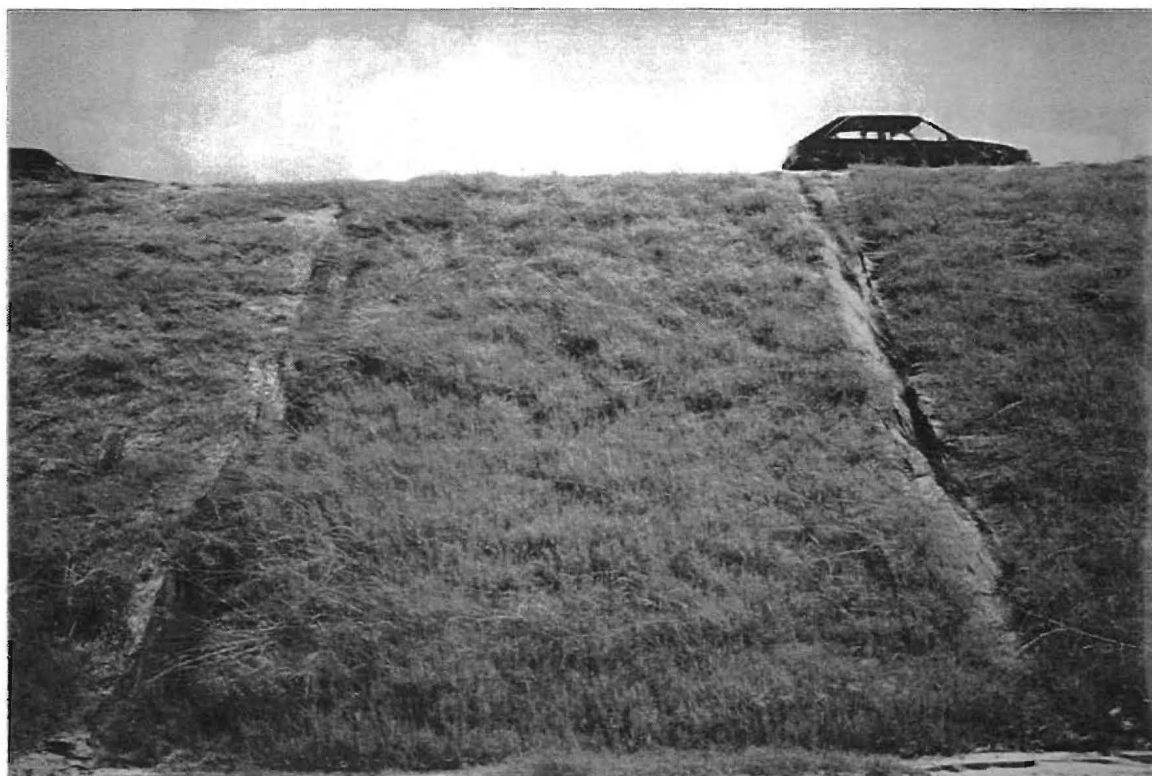
Figure 45. Vegetative coverage on a 3:1 Sand Excelsior product plot
