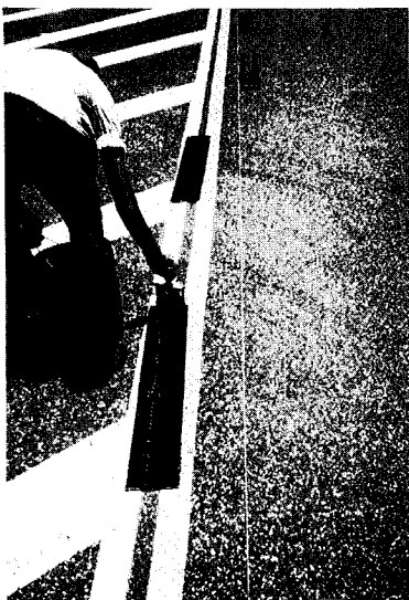
APPLYING MASTIC TO STRIPE
