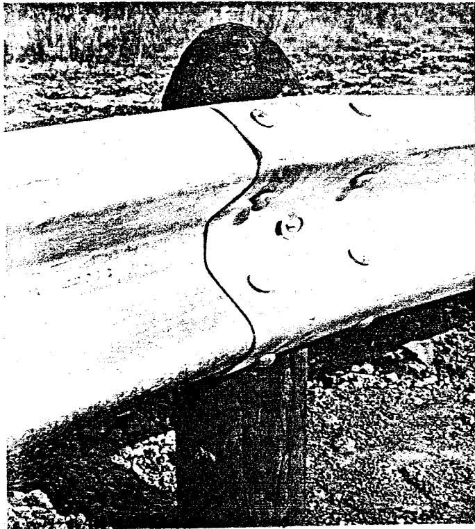
FIGURE 27. | PHOTOGRAPHS OF THE RAIL-POST HARDWARE PRIOR TO TEST 5.
