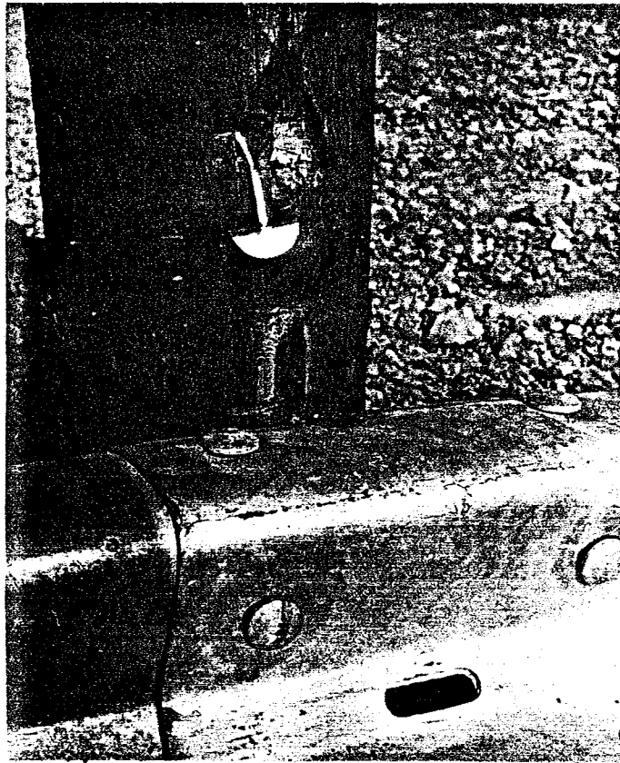
FIGURE 28. PHOTOGRAPHS OF DEPRESSED RAIL POSITION AFTER LOW-SPEED TRIAL TEST.
