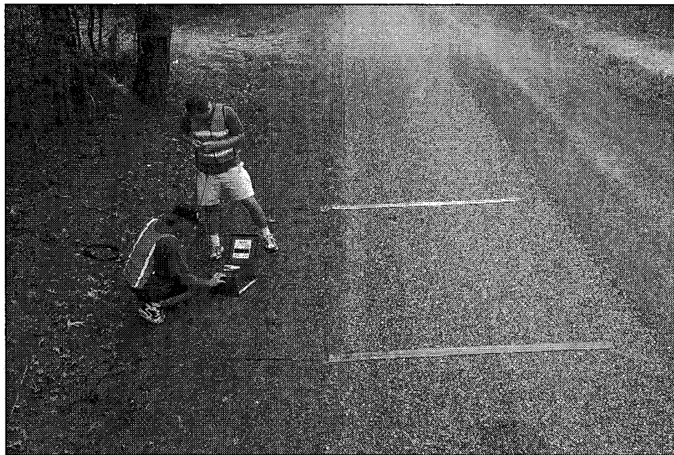
Figure 3-2. Piezoelectric Sensors and Traffic Classifier.
