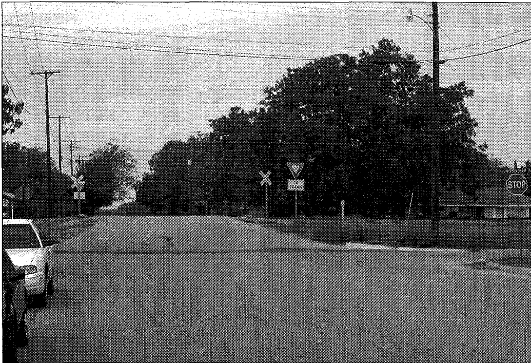
Figure 4-20. Westbound Approach on Oak Street in Wylie, Texas.
