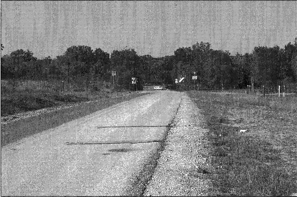
Figure 4-10. Northbound Approach on Farm to Market Road 1748.
