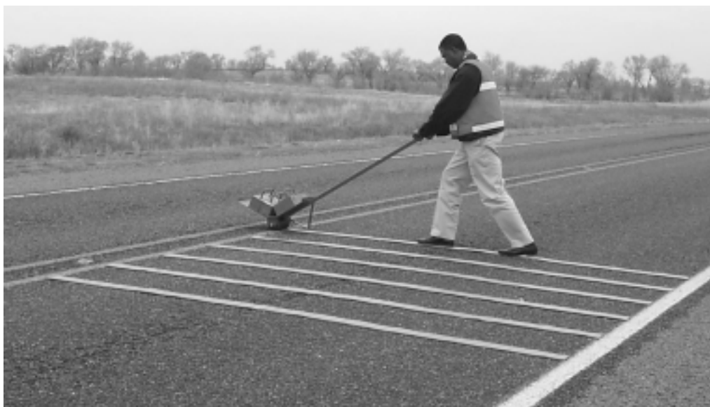
Figure 7. Portable Rumble Strips Installation.
