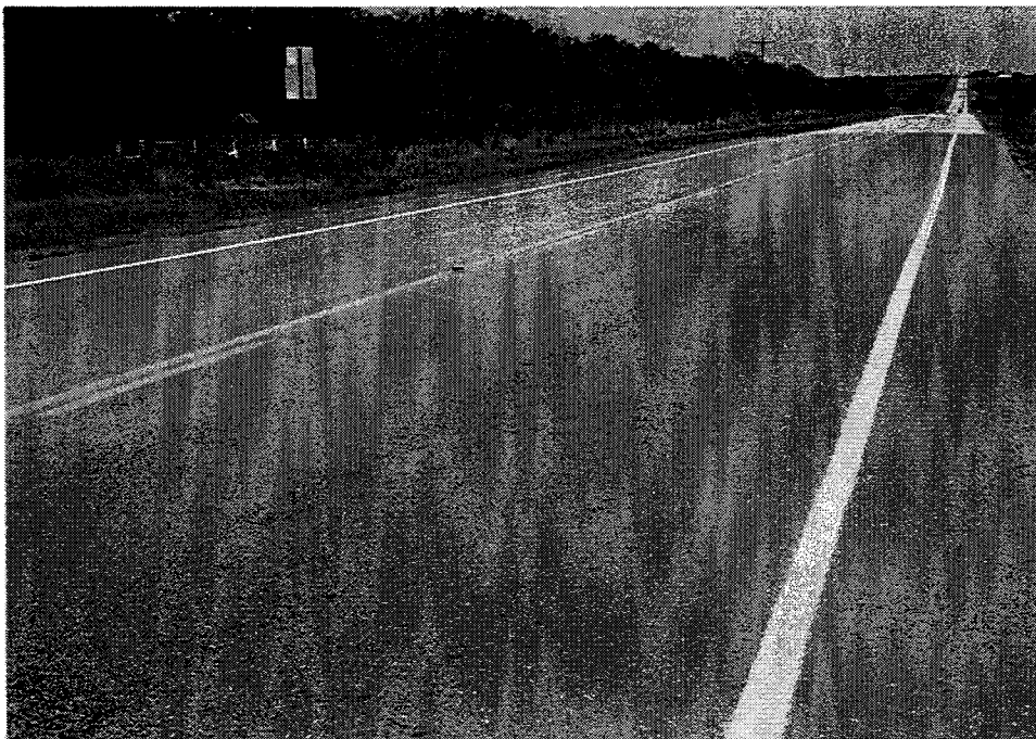
Figure 21. Pleasanton Test Section 5: HMCL/Treated RAP.
