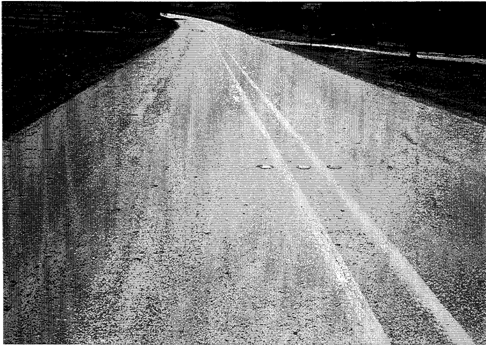
Figure 12. Cleburne Test Section 2: HMCL/Untreated RAP Blend.
