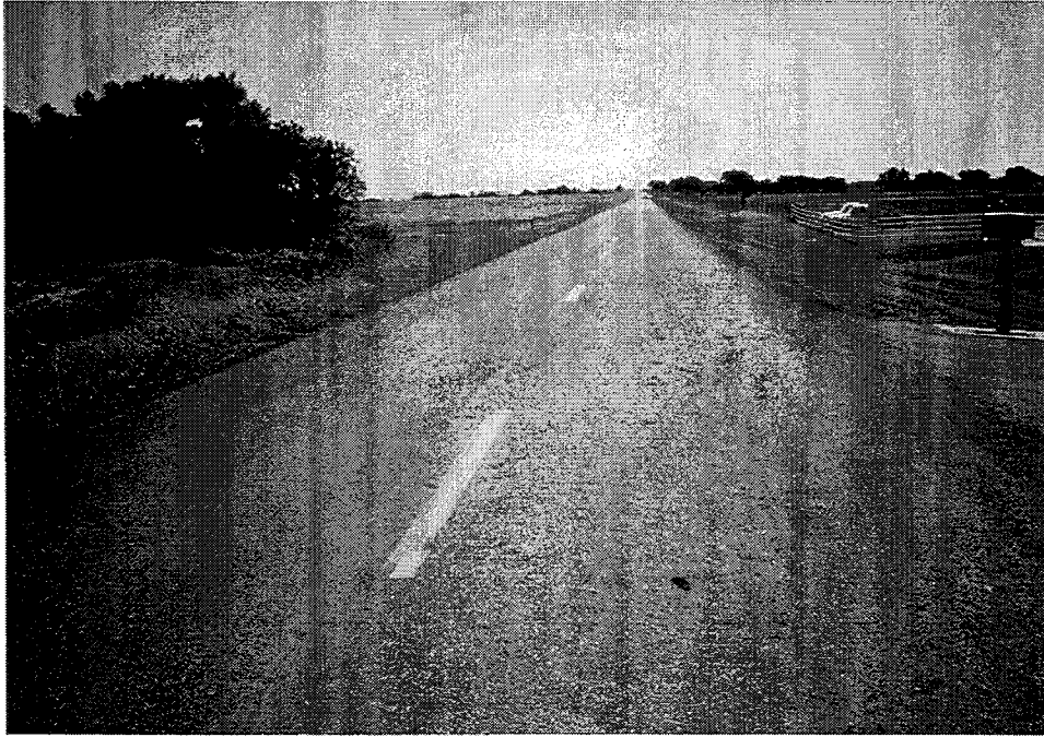
Figure 8. McKinney Test Section 5: LRA/Treated RAP Blend.
