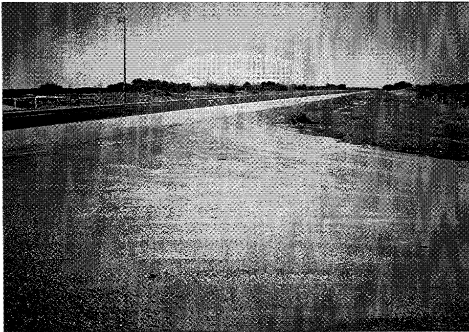
Figure 27. Brownwood County Road Approach.
