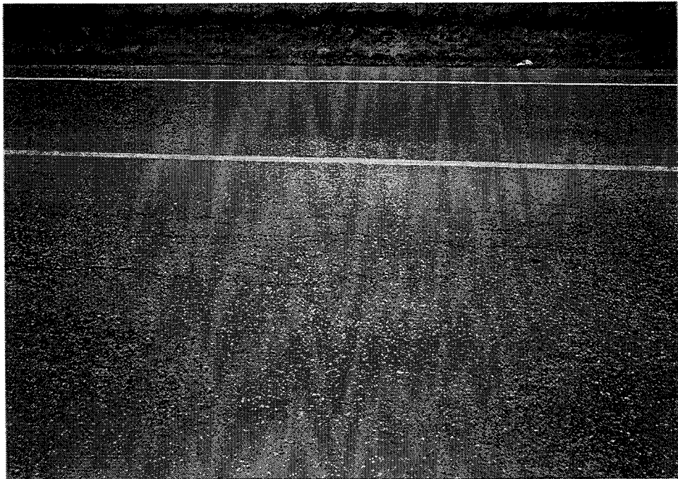
Figure 19. Pleasanton Test Section 3: LRA/Treated RAP.
