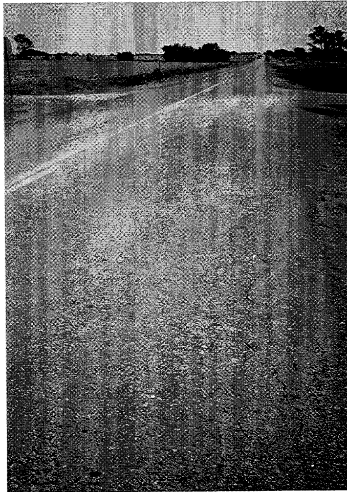
Figure 7. McKinney Test Section 4: LRA/Untreated RAP Blend.
