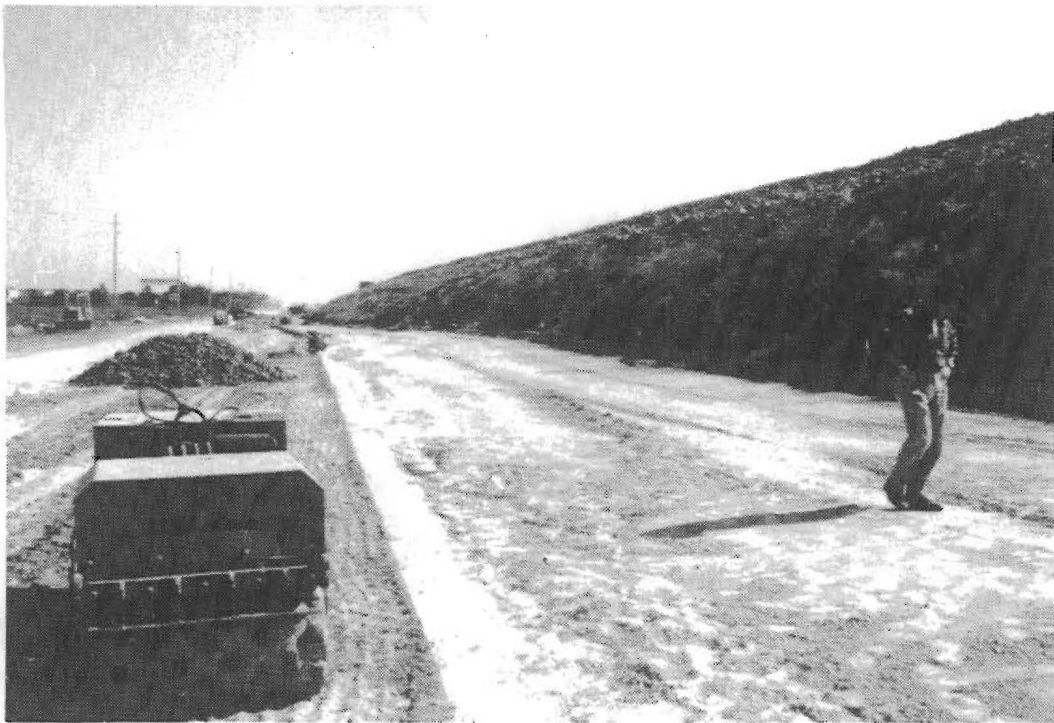
Figure 2.12 Foundation preparation for wall 9
