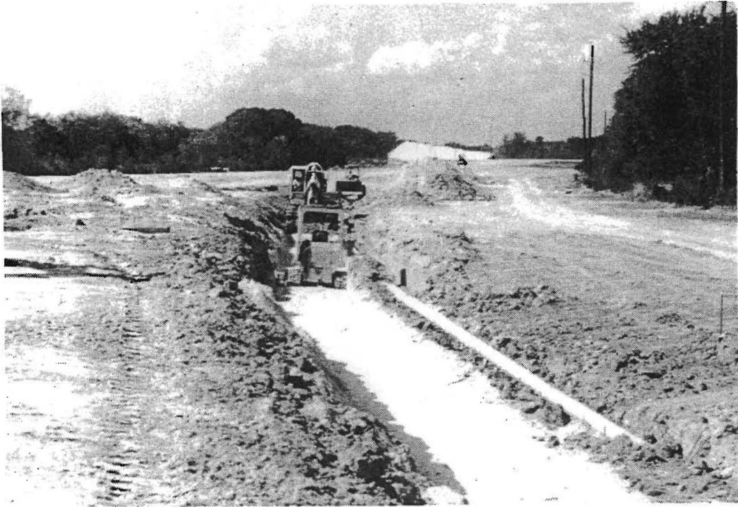
Figure 2.7 Foundation preparation for wall 7
