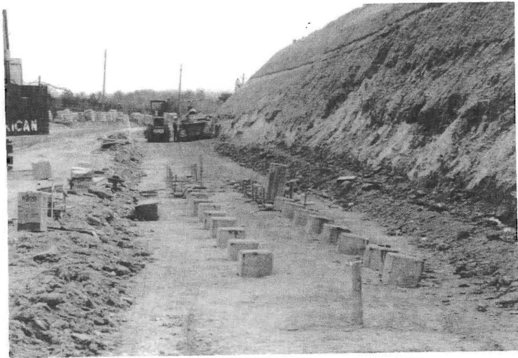
Figure 2.10 Photograph of piled foundation for wall 7
