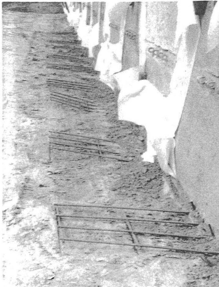
Figure 2.8 Facing panel anchors at wall 7
