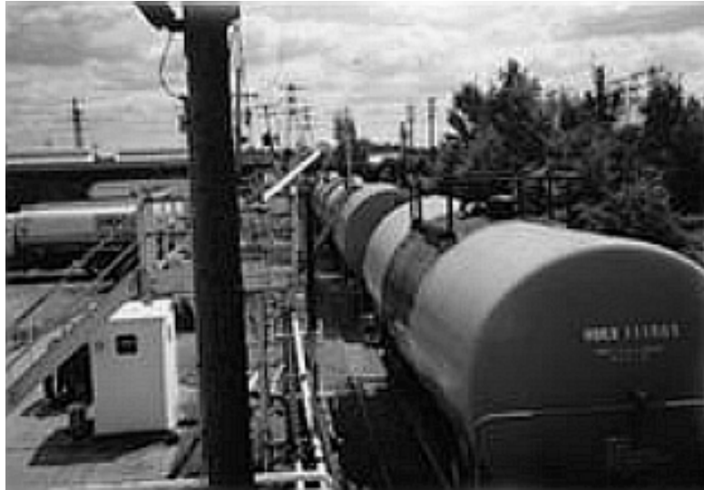
Figure 22: Rail Tank Car Loading Facility (24).
