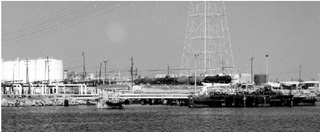
Figure 25: GATX Ship Dock No. 1 at Galena Park Terminal in Houston, Texas. Note Rail Spur and Piping to Storage Tanks.
