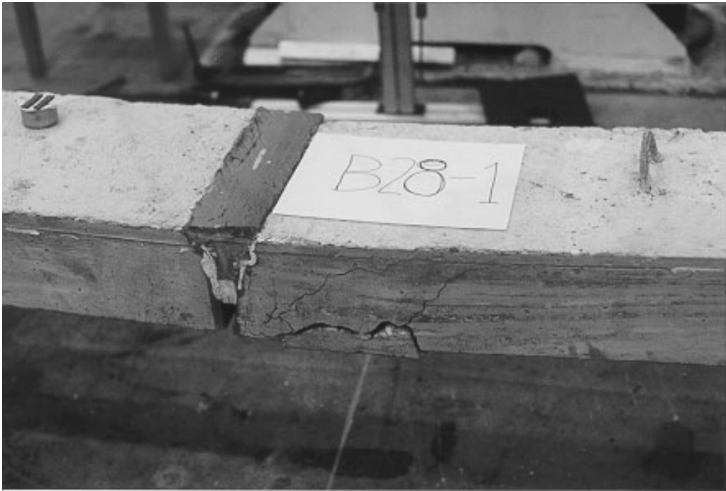
Figure 46. Spalling of Cover Concrete in Beam Connection Test.
