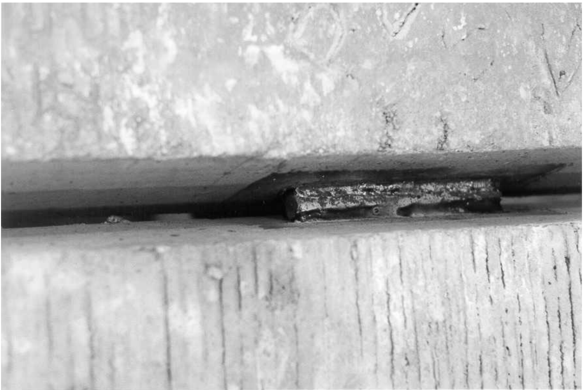
Figure 56. Steel Bar Welded into Connection.
