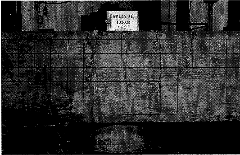
Figure E-9. Specimen 3C Cracking Pattern at P = 160 kips.
