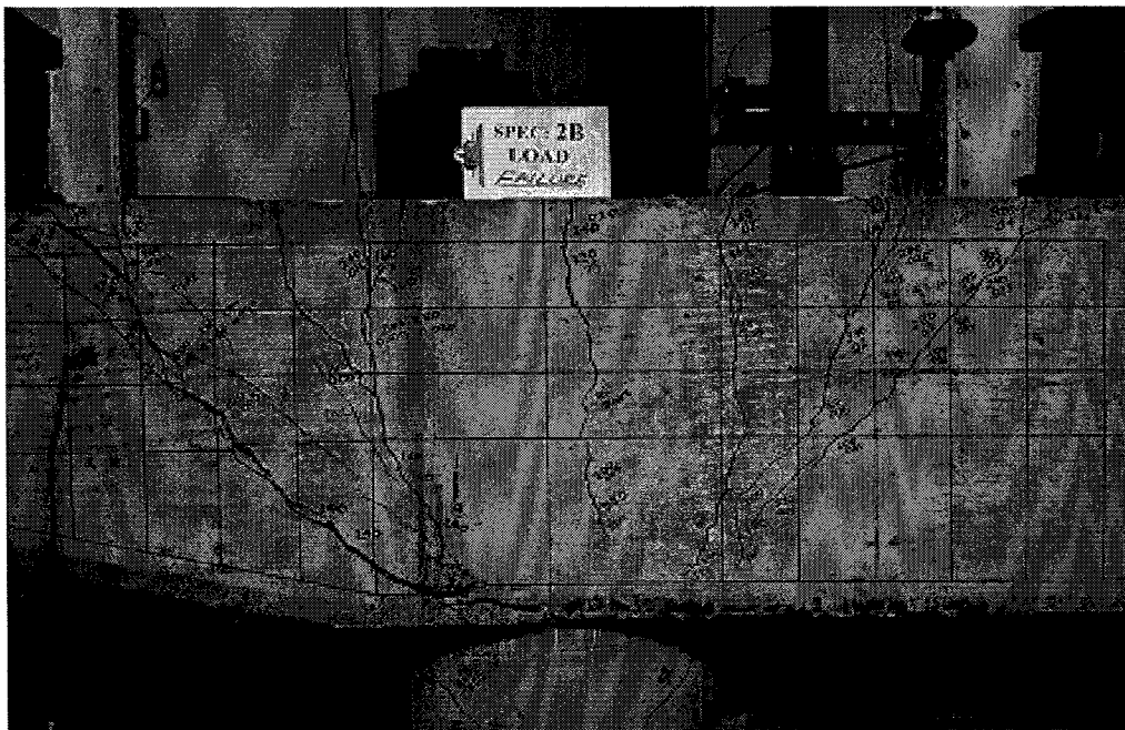
Figure E-8. Specimen 2B Cracking Pattern at P = 390 kips.
