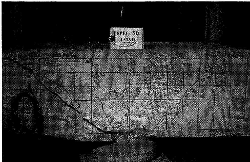
Figure E-18. Specimen 5D Cracking Pattern at P = 470 kips.
