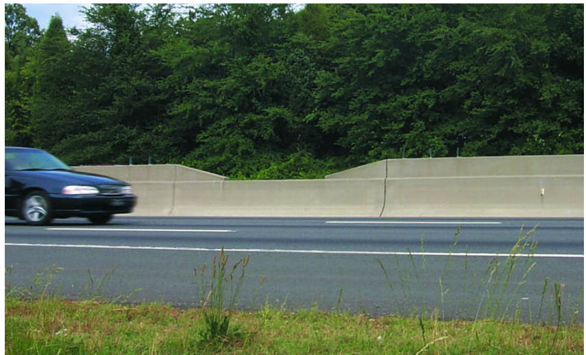
Screening and tall barriers can reduce the negative impact of incidents for opposing traffic.
