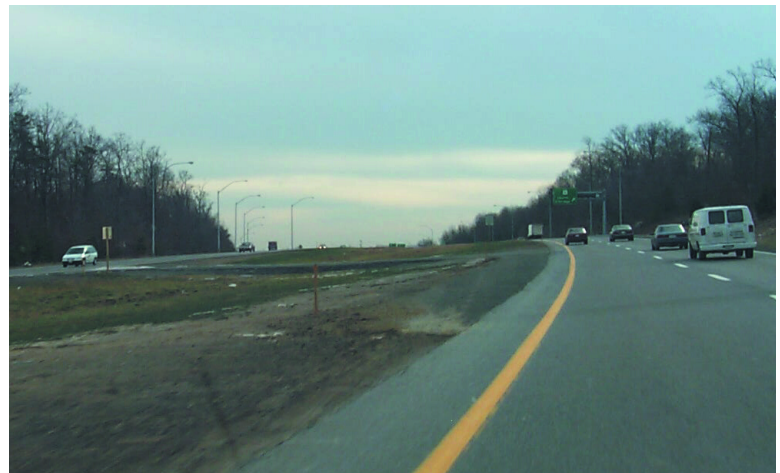
Emergency crossovers can facilitate incident response.
