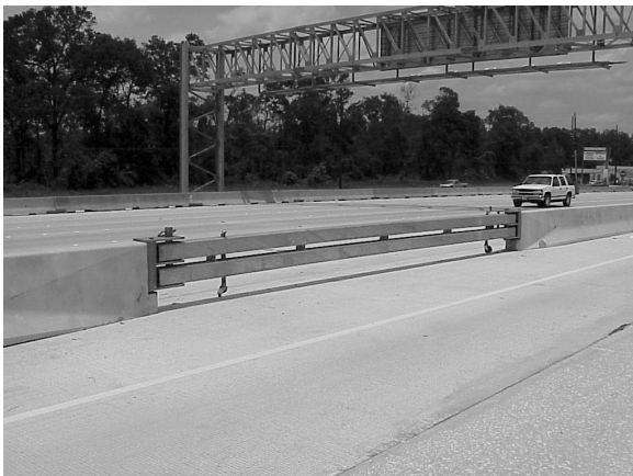
Figure 3-7. TTI Access Gate.
