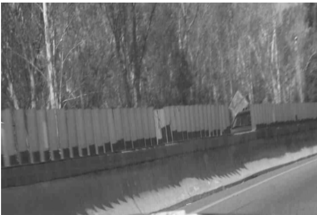
Figure 8-5. Glare Screens in Las Vegas.
