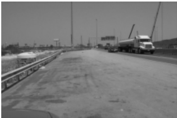
Figure 4-16. AIS Adjacent Construction Site.
