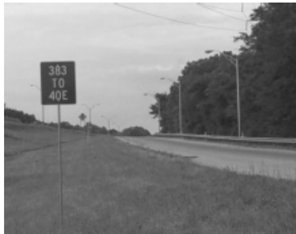
Figure 7-5. Ramp Marker Sign in Tennessee.
