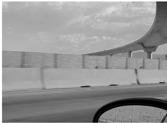
Figure 8-4. Temporary Glare Screen.
