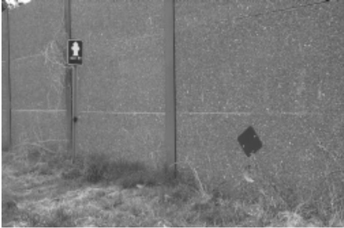
Figure 9-5. Fire Hose Opening and Sign.
