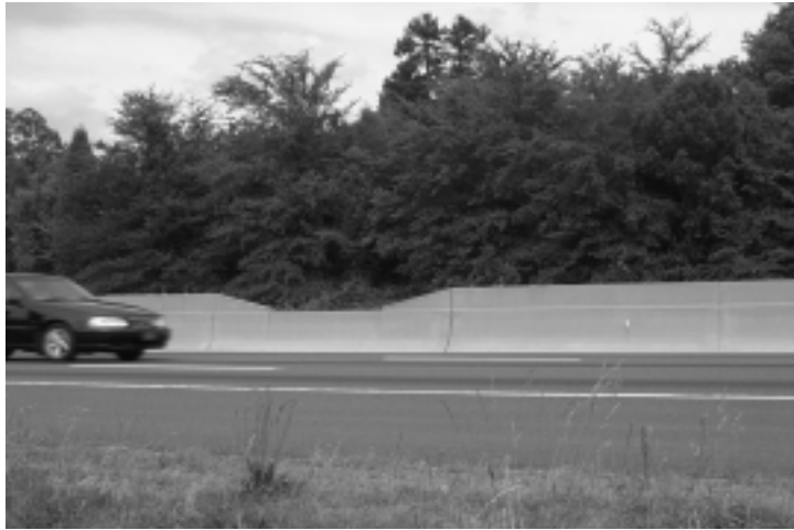
Figure 8-7. Concrete Barrier Opening in Charlotte, NC.
