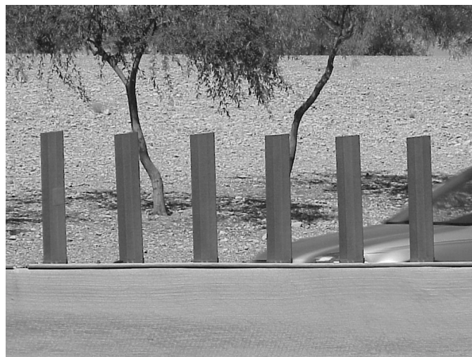
Figure 8-1. Glare Screen on Concrete Barrier.
