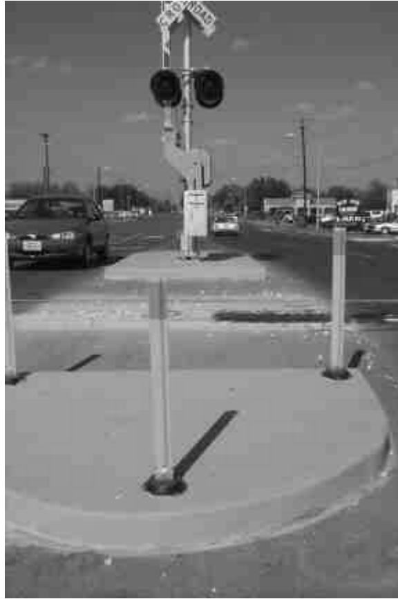
Figure 6. Gate Arm Located in Median on Raised Island.
