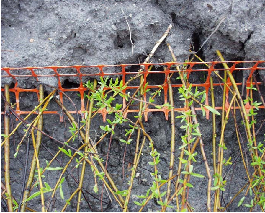
Figure 18. Cuttings Separated by Plastic Net.
