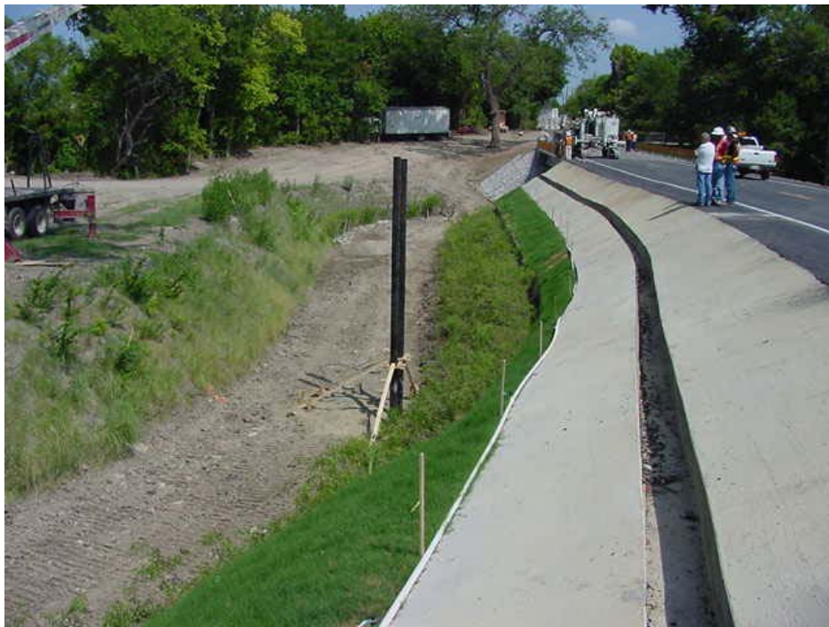
Figure 12. Drainage Flume Along Goode Road.
