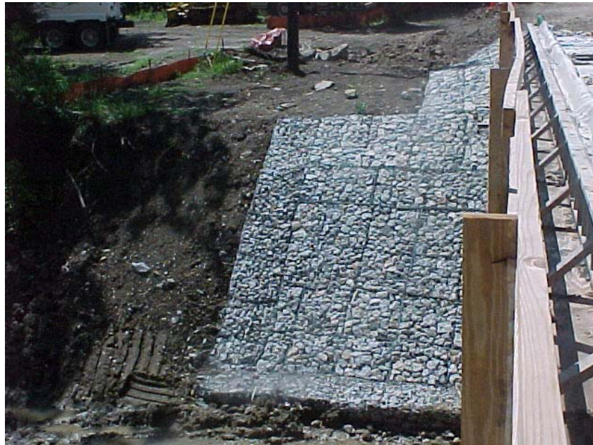
Figure 6. Gabion Mattresses.
