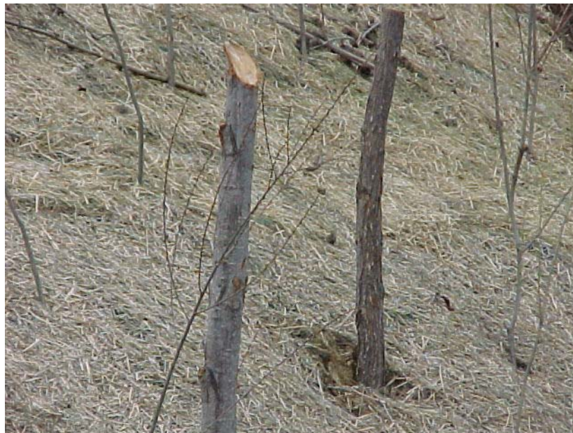
Figure 11. Installed Dormant Posts with Erosion Control Blankets.
