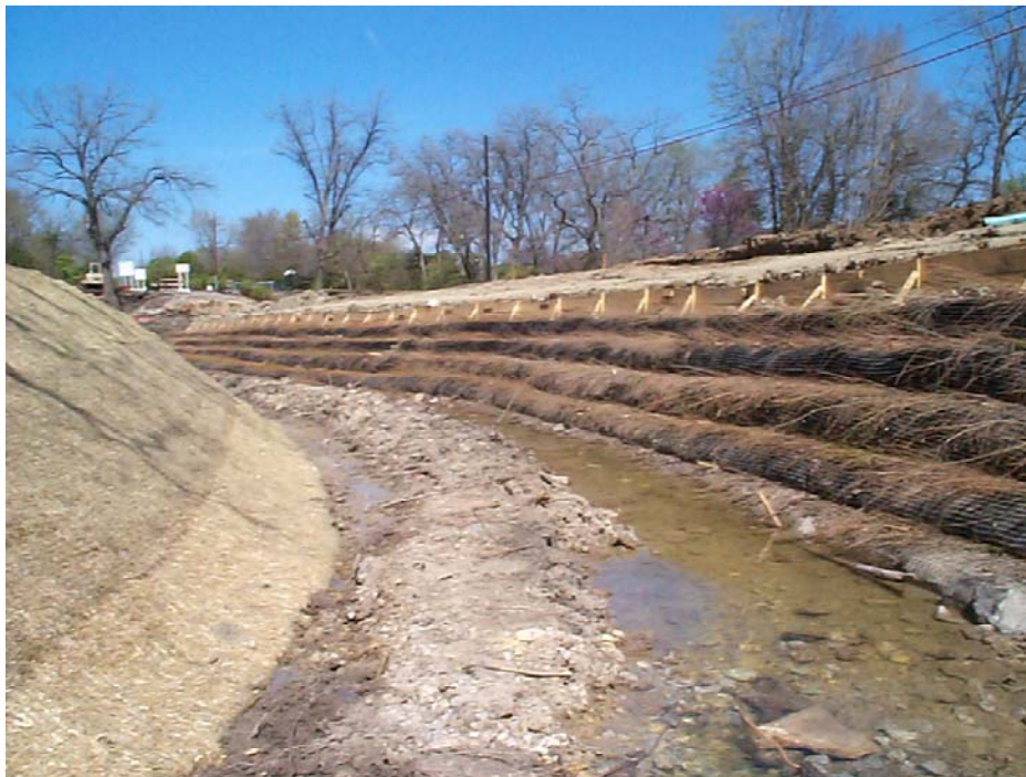
Figure 9. Installed Vegetative Geogrids in March 2001.
