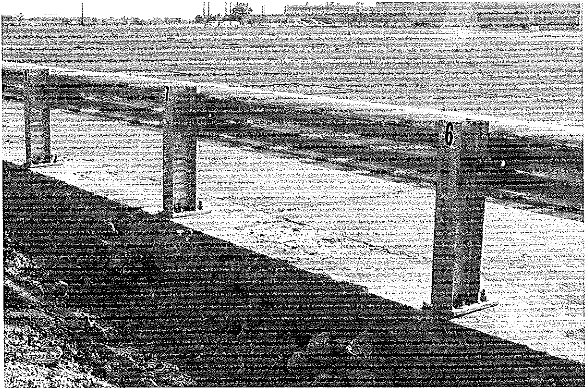
Figure 2. Texas Type T6 Bridge Rail Installation before Test 418048-2
