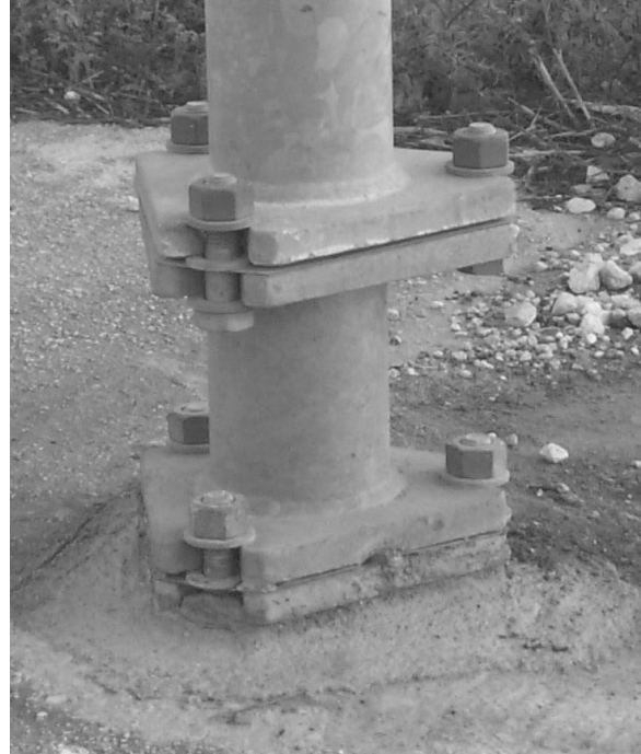
Figure 3. Slip Base Extension.
