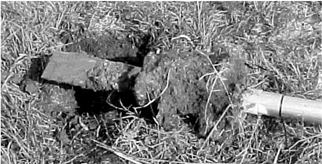
Figure 2. Contractor Partial Concrete Foundation.
