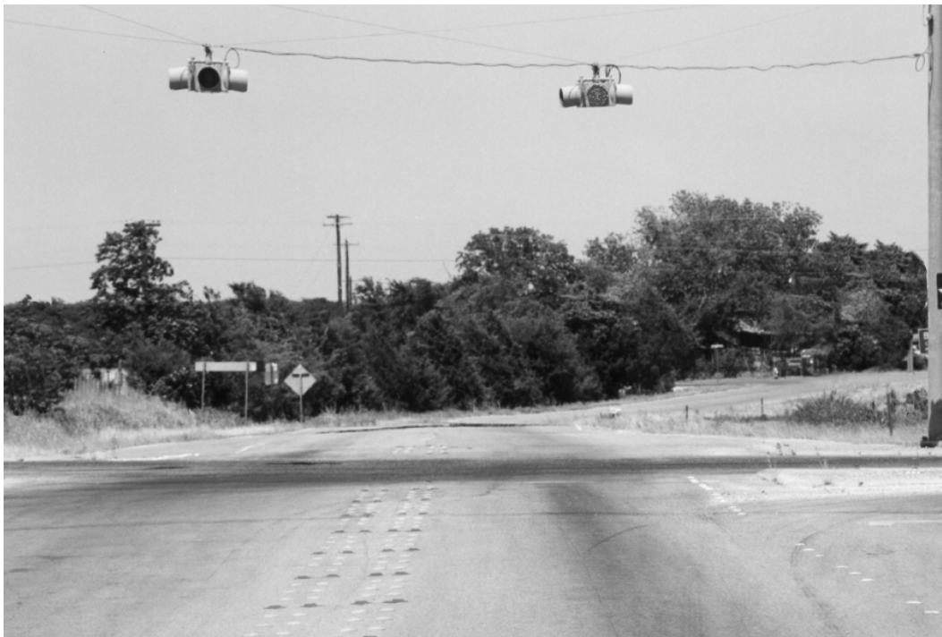
Figure B-6. Flashing Red Intersection Beacon (Survey Question #6).
