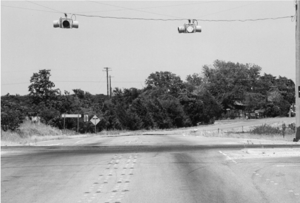
Figure B-3. Flashing Yellow Intersection Beacon (Survey Question #3).
