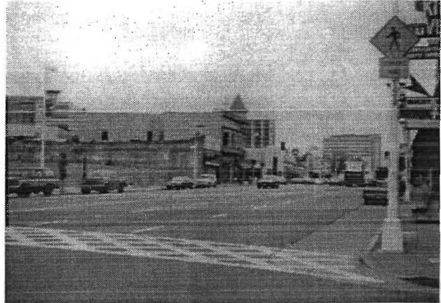
Figure 4-10. Lattice Crosswalk Markings in Oakland, CA.
