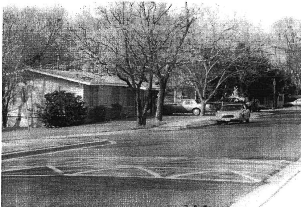
Figure 2-1. Speed Hump in Austin, TX.
