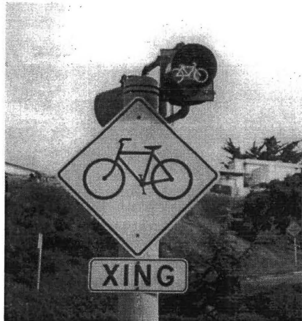
Figure 5-40. Flashing Bicycle Beacon in Monterey, CA.
