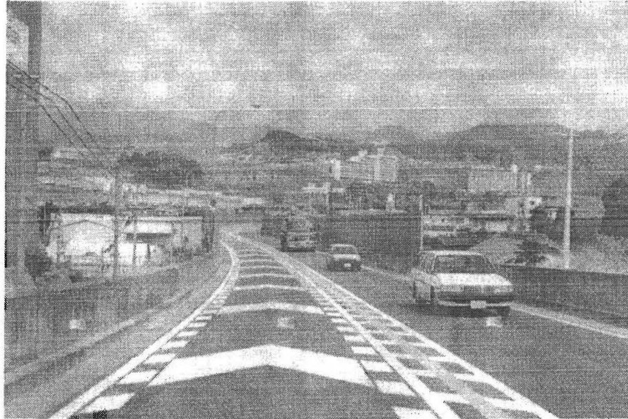
Figure 4-27. Converging Chevron Pattern on Route 371, Kawachinago Bypass, Japan. (12)
