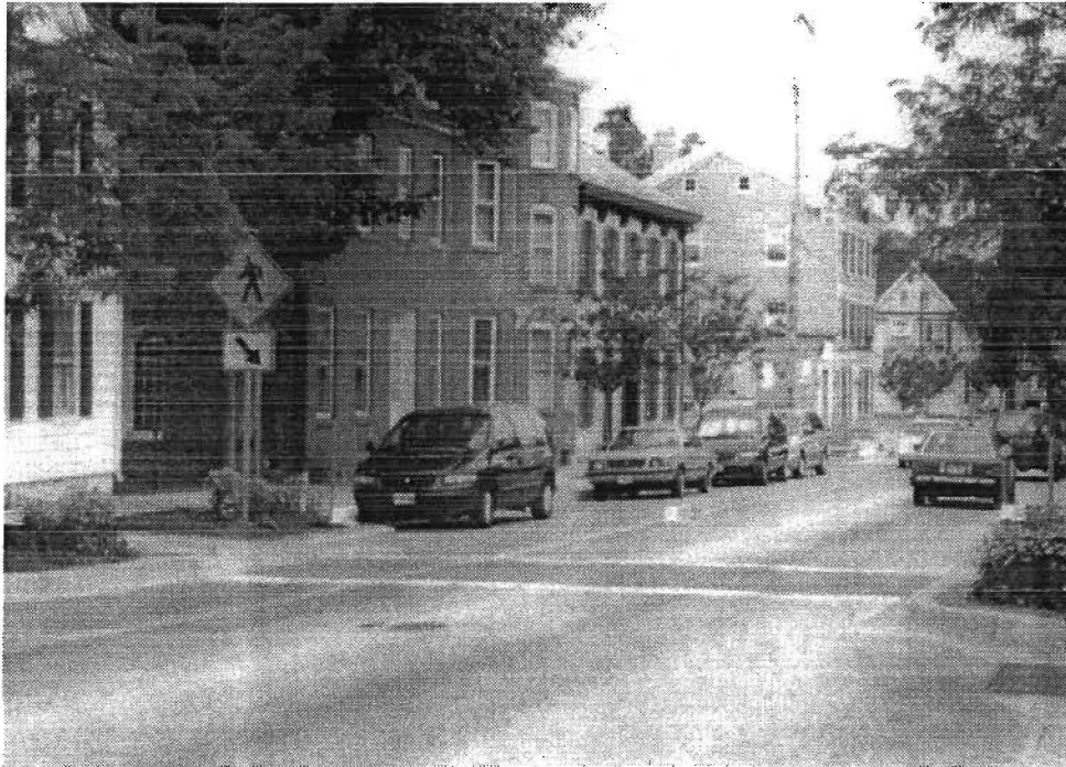
Figure 3-4. Neckdown with Brick Crosswalks, Landscaping, and Parking in Westminster, MD.
