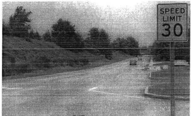
Figure 5-8. Speed Limit Sign in Montgomery County, MD.
