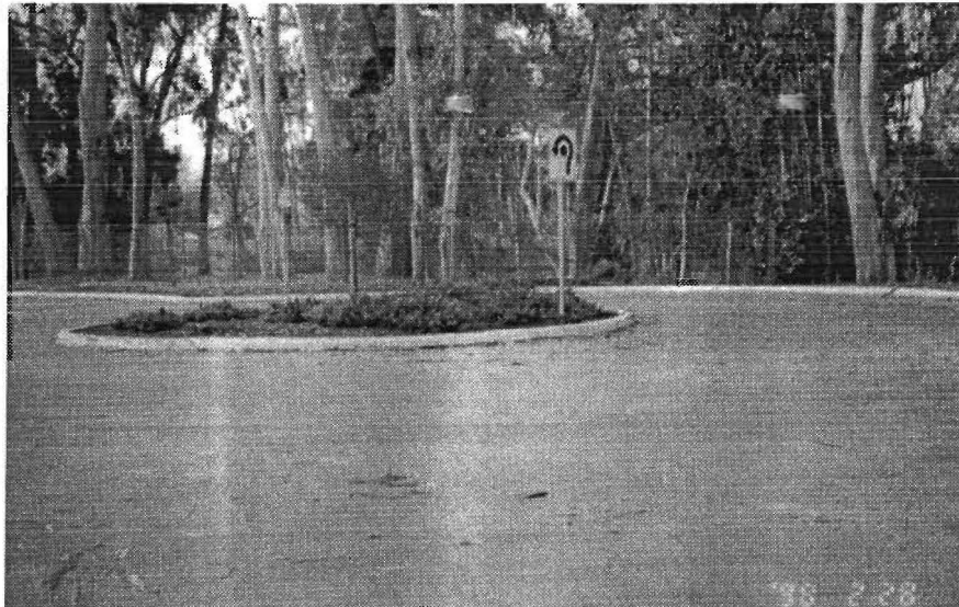
Figure 3-40. Traffic Circle in Monterey, CA.
