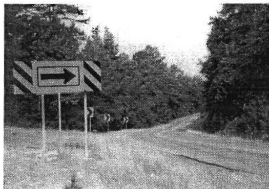
Figure 5-14. Curve with Signs and Pavement Markings in East Texas.
