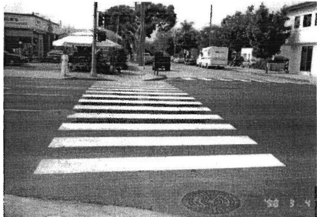
Figure 4-12. Ladder Style High- Visibility Crosswalk in Santa Barbara, CA.
