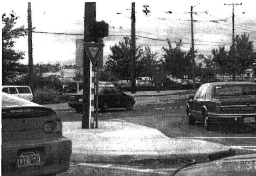
Figure 3-30. Forced-Turn Island in Montgomery County, MD.
