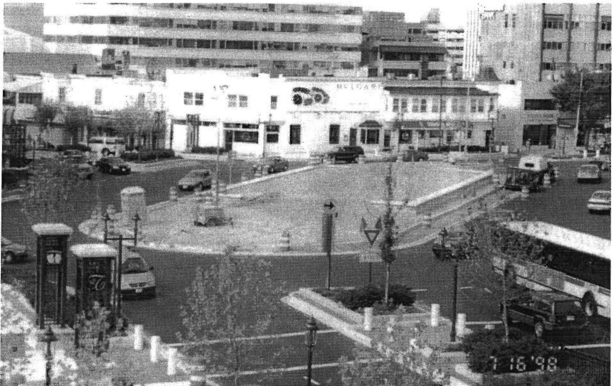
Figure 3-53. Oval Roundabout Under Construction in Towson, MD.
