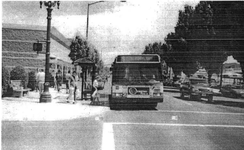
Figure 3-6. Bus Stop at a Neckdown (also known as a Bus Bulb) in Seattle, WA.
