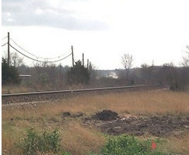
Note railroad track curving toward the left
