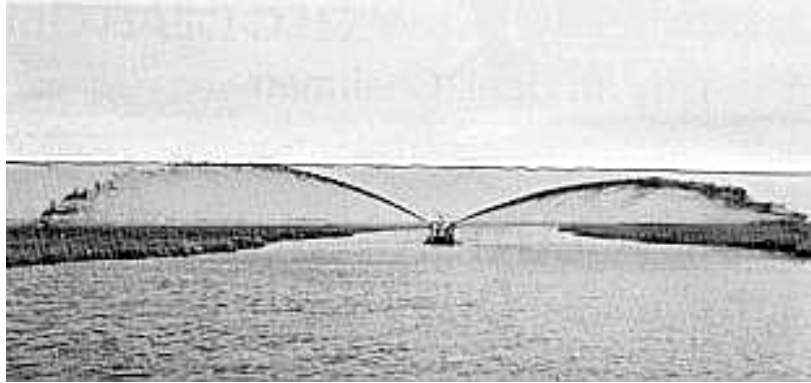
Figure 3-14. Thin-Layer Disposal from a Channel through a Wetland (Deal, 1998).
