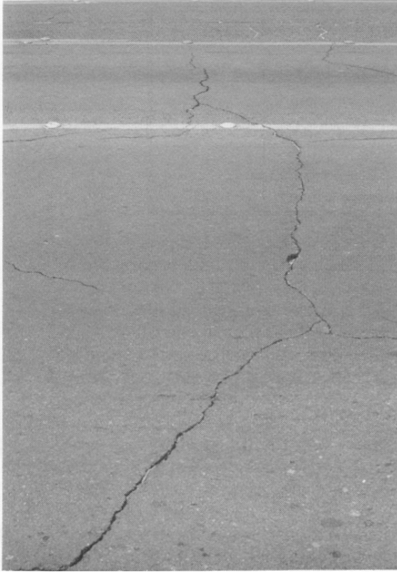
Figure 1. Examples of Transverse Cracking (TxDOT, 1998).
