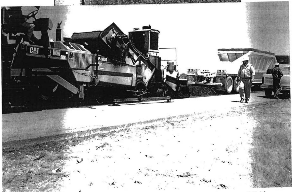
Figure 13. Lay Down Operation Large Stone Superpave Mix on IH 20.
