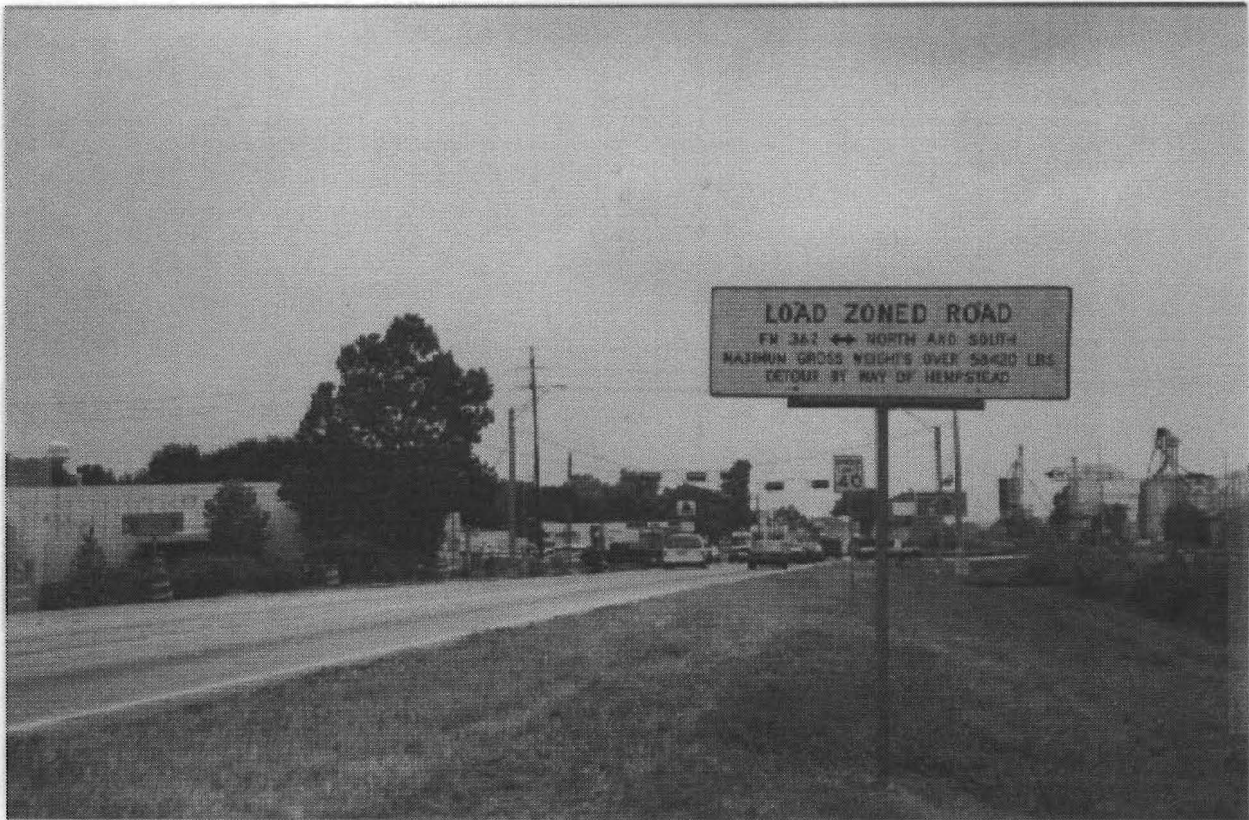
Figure 1. Sign for a Load Zoned Segment of FM 362 (GVW 260 kN).
