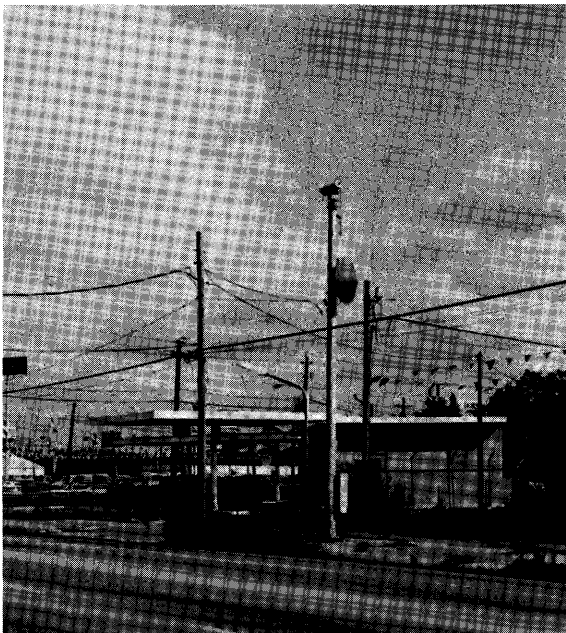
TELEVISION CAMERA AND MICROWAVE TRANSMITTER INSTALLATION AT WAYSIDE DRIVE AND TELEPHONE ROAD
