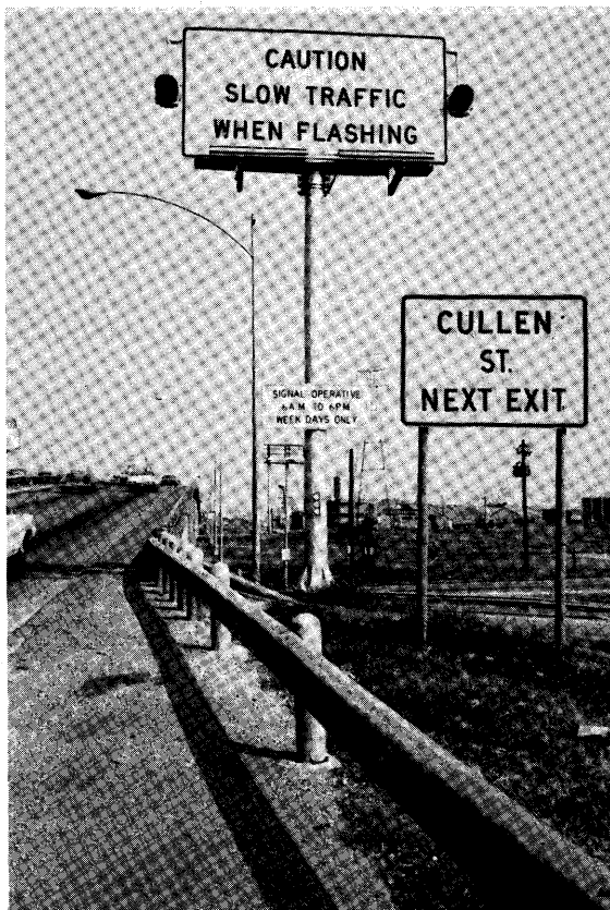
Figure 1 - Warning Sign with Flashers
