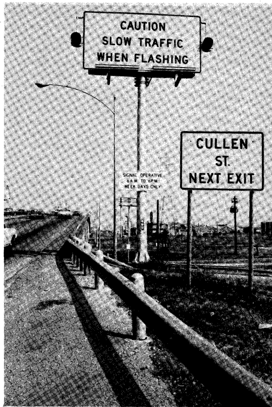
Figure 3. Warning Sign with Flashers
