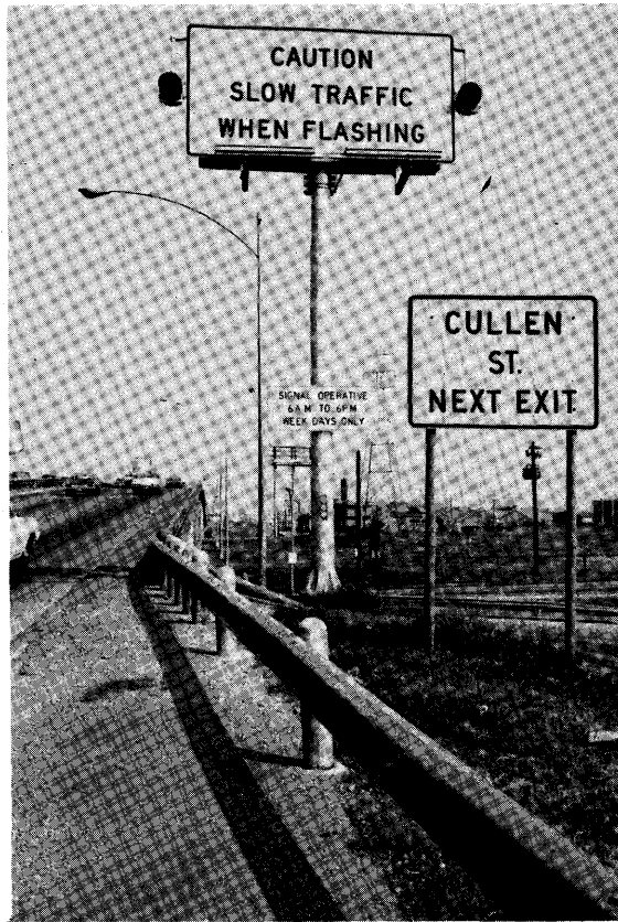
Figure 1 - Warning Sign with Flashers
