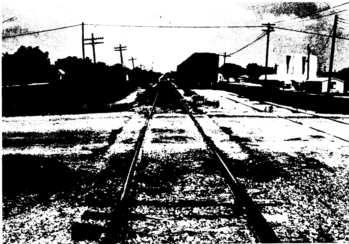
FIGURE 8.- A HIGHWAY-RAILROAD GRADE CROSSING IN HOLLAND, TEXAS WITH ITS TYPICAL DIFFERENTIAL PERMANENT DEFORMATION BETWEEN RAILROAD AND ADJACENT PAVEMENT STRUCTURES
