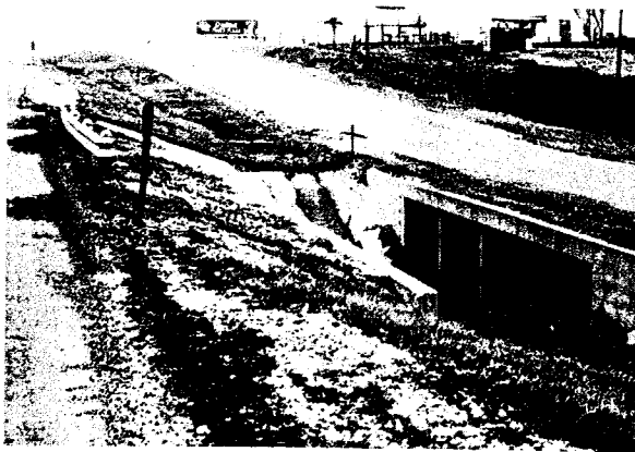
c. Gap between Culvert Headwalls on Parallel Roads (Code 09-02)
