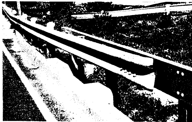
b. Shop Fabrication--Develops Full Beam Strength
