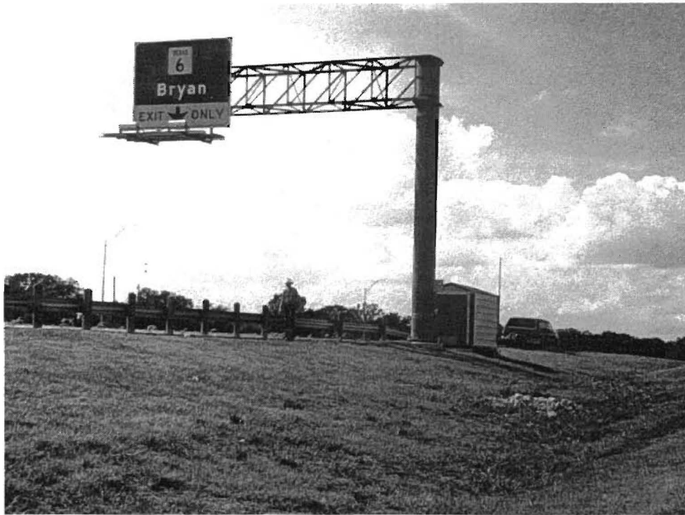
FIGURE 8 Photograph of COSS field study structure near Hempstead, Texas.
