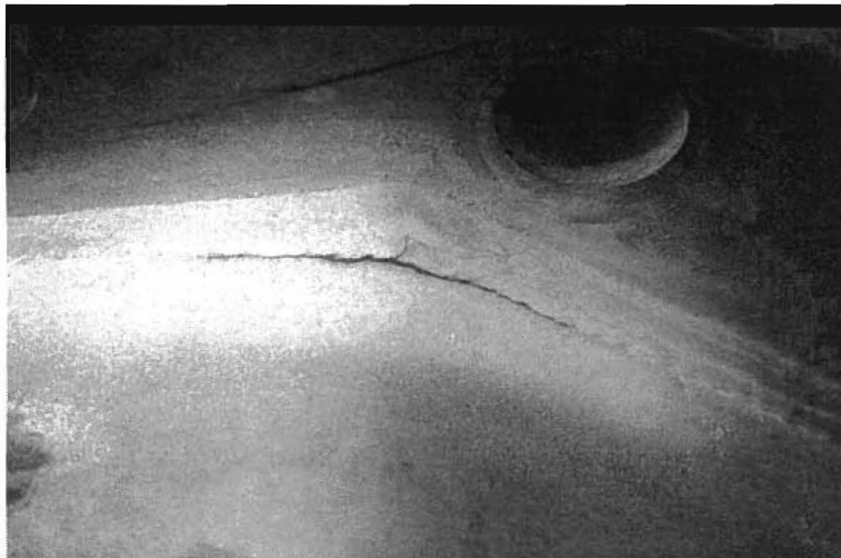
FIGURE 85 Photograph of fatigue crack adjacent to bolt L in HMIP 4 1/2 UNC laboratory specimen.
