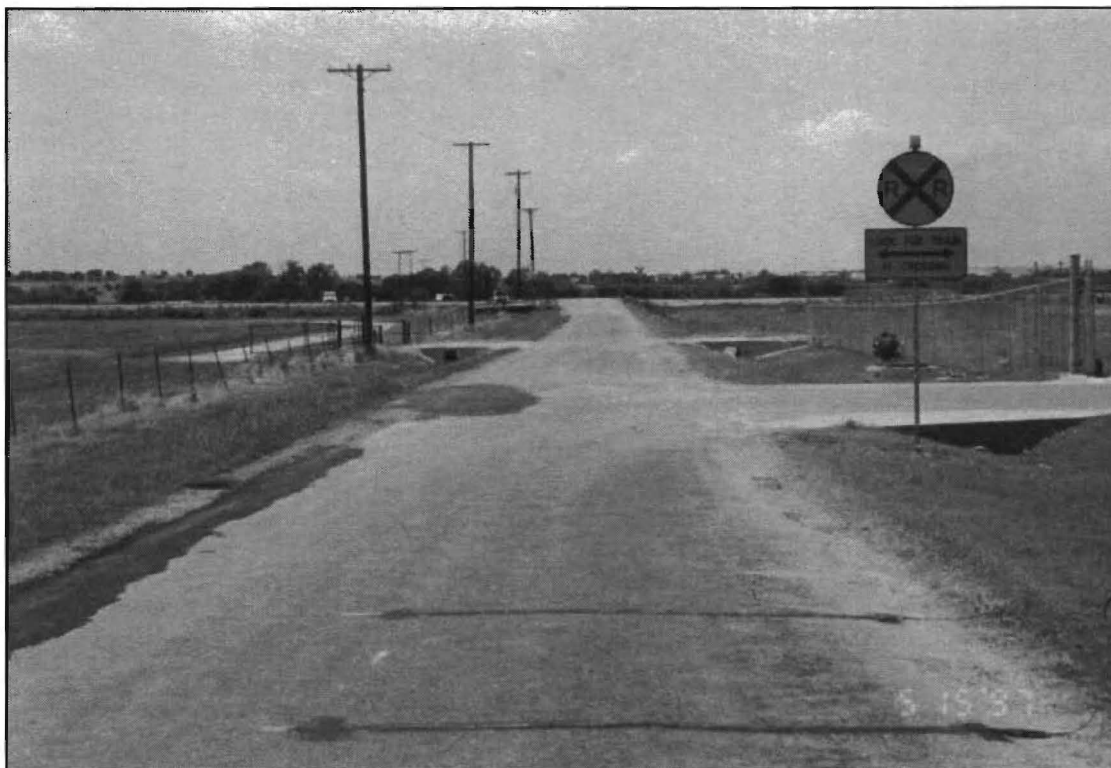
Figure 2.7. Completed Experimental Set-Up on East Approach
