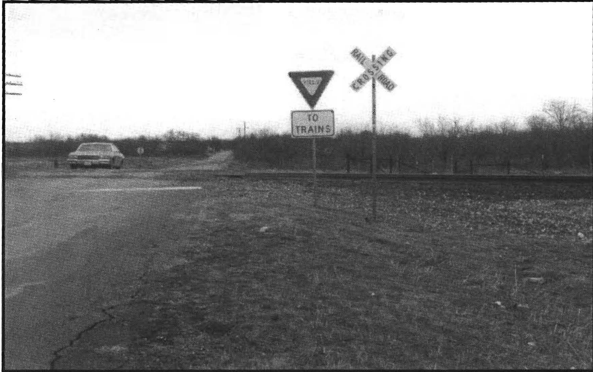
Figure 4.2. The YIELD TO TRAINS Sign System Installed at a Test Crossing
