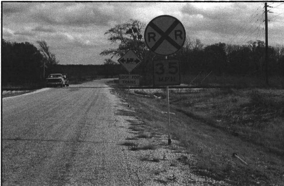
Figure 4.3. The LOOK FOR TRAINS Sign System Installed at a Test Crossing
