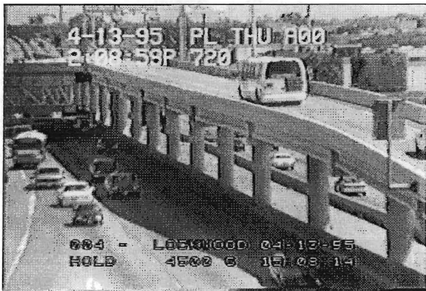
FIGURE 3. HOV Lane T-Ramp Blocking View of Far-Side Freeway Lanes
