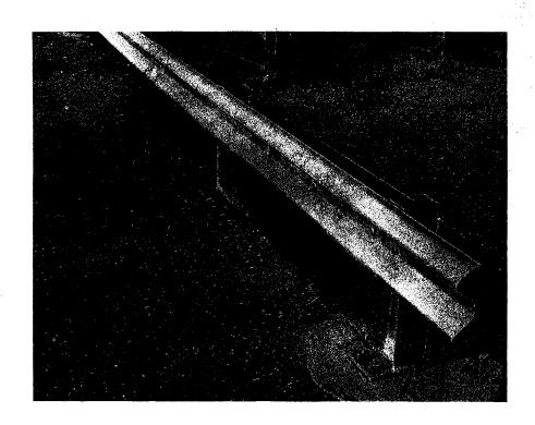
Figure 22, Guardrail Anchorage Behind Rigid Wall.
