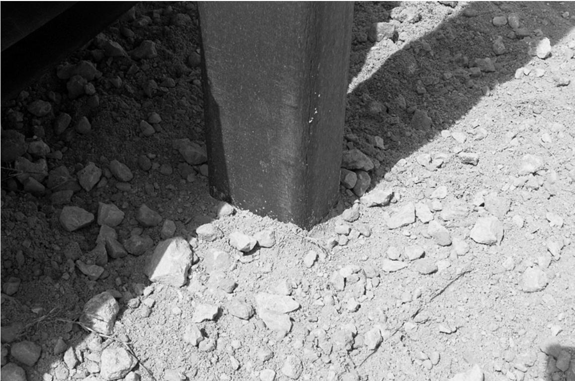
Figure 39. Recycled Plastic Sign Support Before Test 414588-3.
