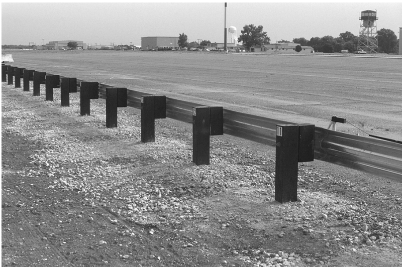
Figure 48. Plastic Post W-Beam Guardrail Installation Before Test 414588-1.
