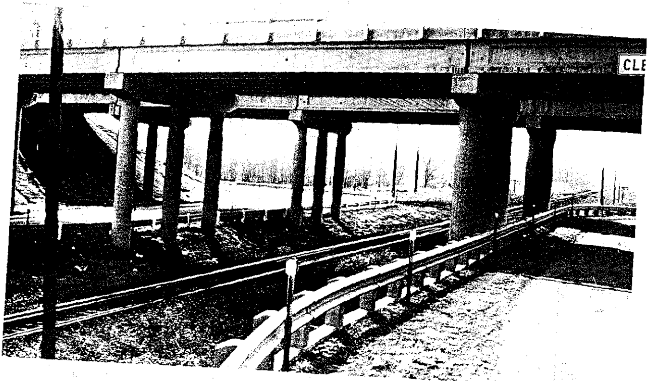
Figure 1. St. Louis-San Francisco Railroad Overpasses.
