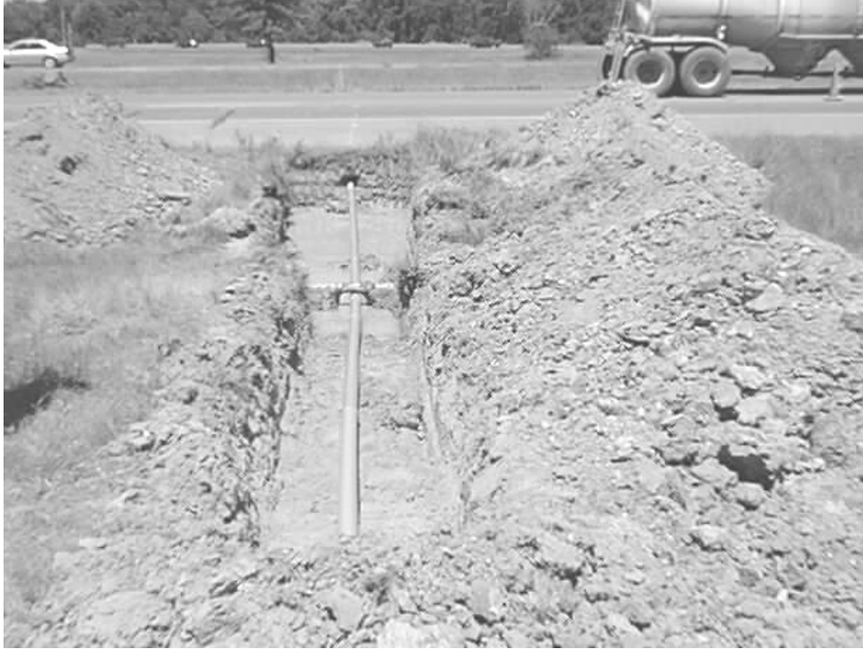
Figure 3. Installation of Microloop Conduit under SH 6.
