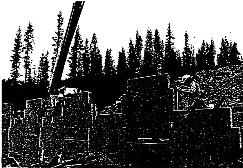
Figure 4.12 Placement of the second row of wall panels and the associated support or bracing for the panels.
