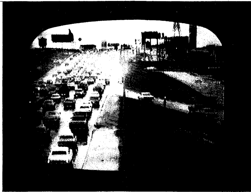
CCTV Surveillance of Ramp Metering System
