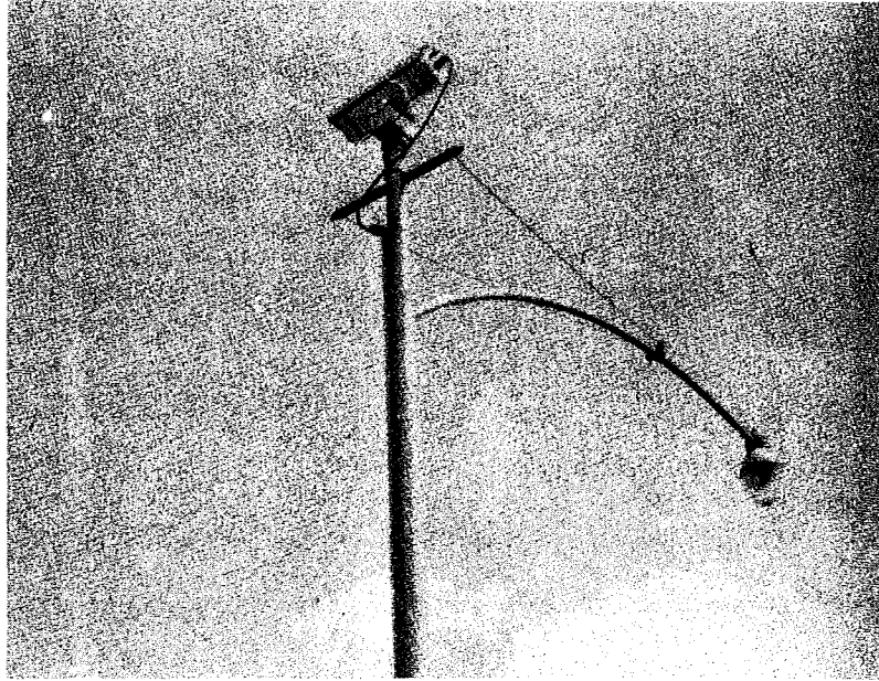
Camera Installation on Existing Luminaire Pole
