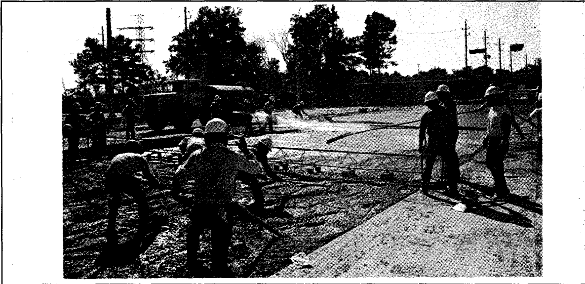
Figure 5. The Impact of an Improperly Managed Accelerator on Finishing Operations.
