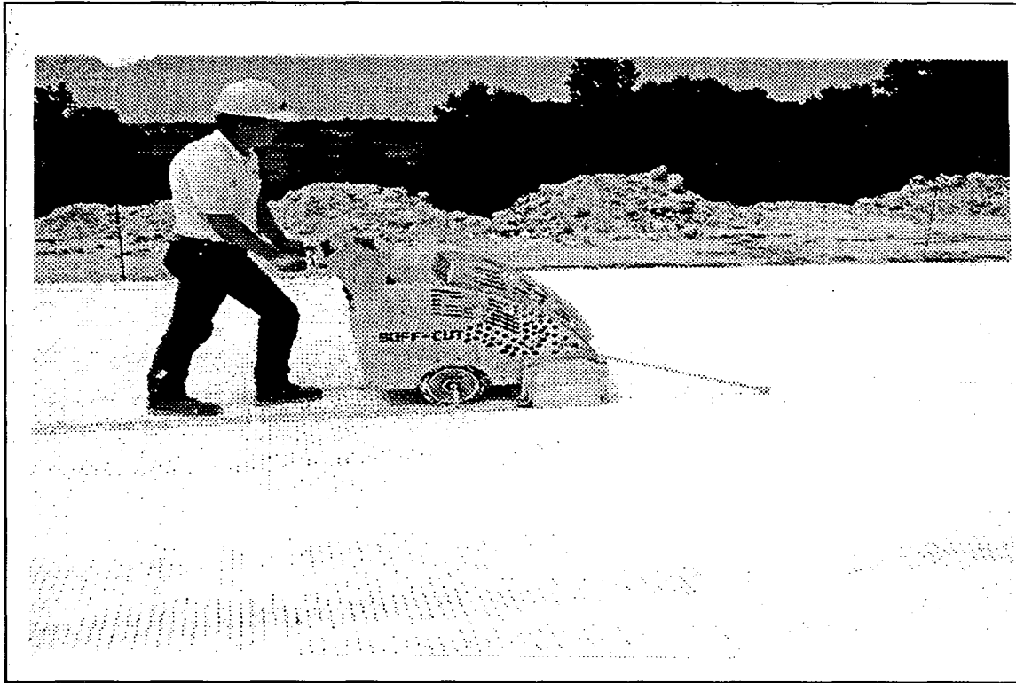
Figure 30. Soff-Cut Early Age Sawcutting Machine.
