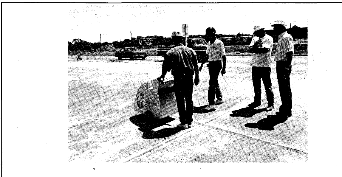
Figure 8. An Example of Early-Aged Sawcutting.
